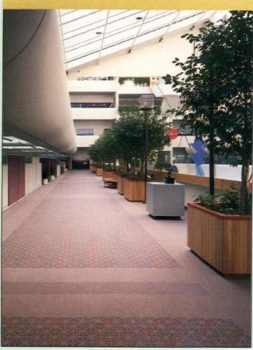
Atrium skylight pours light into interior of building where light scoops shunt illumination where needed—a power-saving concept.
