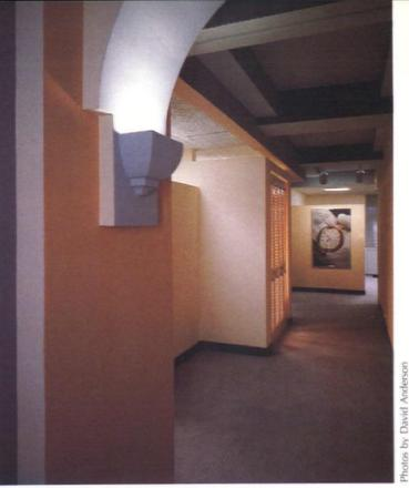
Unsightly plumbing shafts are transformed into gracious design elements used to support full- and half-arches, adding variety to interiors for Channel 13/WNET, N.Y. headquarters planned by Colbert deSign.
