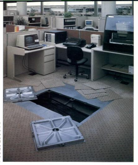
As flatwire systems and other space-saving electrical delivery methods gain credence in the marketplace, access floors are expected to increasingly handle distribution of non-electrical services, such as task air. Shown to right is Donn's steel-panel system which is pumped with cement mixture to assure wearability and reduced sound.
