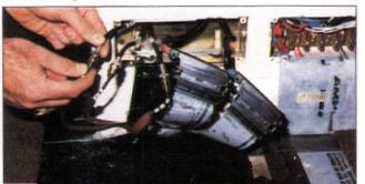
Shown is AMP's combination floor-mounted transition fitting which handles both power circuits,(left) and telephone circuits,(right) Metal shield provides a barrier; steel cover is in background.
