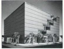
Photo of 500,000 sq.-ft. Houston Design Center model illustrates diagonally-stepped, 10-story atrium which forms a central circulation canyon.
