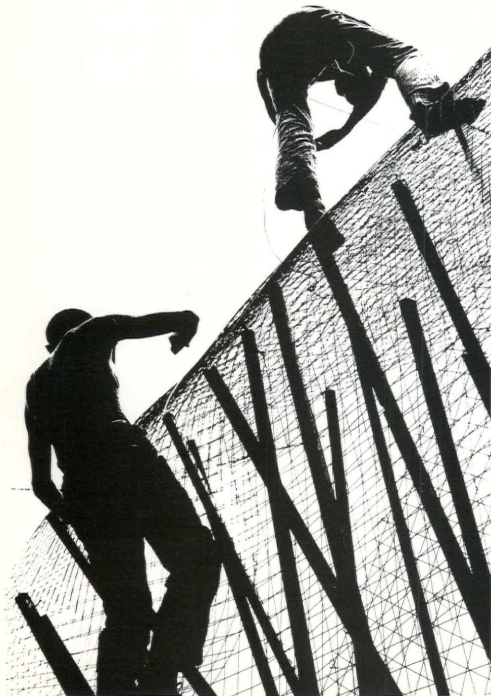
Volunteer builders, left, secure wire mesh framework to temporary wood supports. After mesh is coated with mortar, it will be self-supporting. Above, physical phenomena on which the design has been based: 1, Moebius strip, a "one-sided" figure; 2, Klein bottle, with interior merging into exterior; 3, asymmetrically curved beam.
