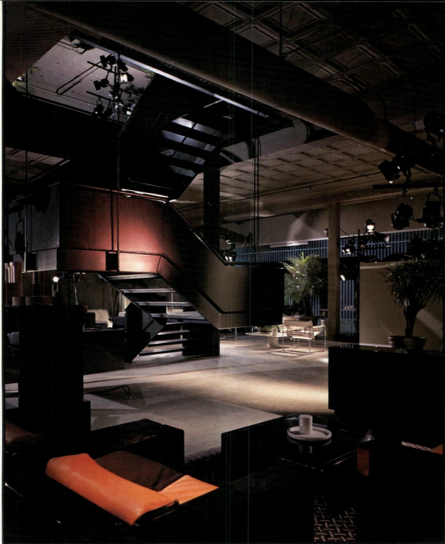
Open-tread stair is suspended from second floor by eight 3/4" steel rods. Original pressed tin ceiling has been retained.
