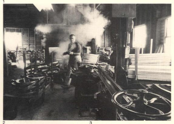
Out of the super-heated steam oven (1) and into the special jig for forming seat frames comes the wood, now ready for bending. Super-steamed dowel for bentwood chair is removed from oven (2), affixed to jig (3), bent into place (4), and clamped for drying overnight (5). Parts come together in this classic bentwood chair (6), one of 23,000 produced annually in Thonet's U.S. plants.
