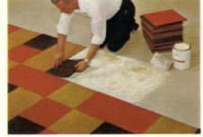
**Easy to install.** Ozite adhesives do the job in a jiffy. Tiles are easy to cut with a knife or scissors. Can be installed in sections. Damaged tiles can be easily replaced by maintenance people. Ozite Carpet Tiles are ideal for hotels, motels, schools, stores, hospitals—all residential and commercial installations. They provide softness, warmth and acoustical value hard-surface tile can't give.
