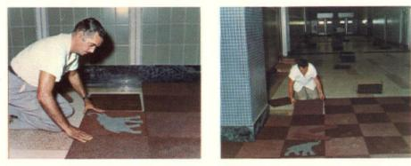
Loose-laid Heugaflor carpet squares quickly go in place without adhesives or time wasting measuring or tacking.
