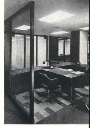
Since no underfloor ducts existed in the sales area, the designers solved the problem by using the base of the center run of storage cabinets (above and below) as a raceway to feed electrical outlets, telephones and Telequote cables. Partitioned columns (section above) also serve as ducts for electrical lines.
