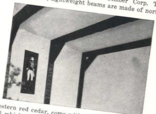
western red cedar, come with a factory-routed channel which is secured over a furring strip with finishing nails. The beams, in 4 by 5, and 2 by 6 inch sizes, are available in standard lengths from 8 to 24 feet, in 2 inch increments.
