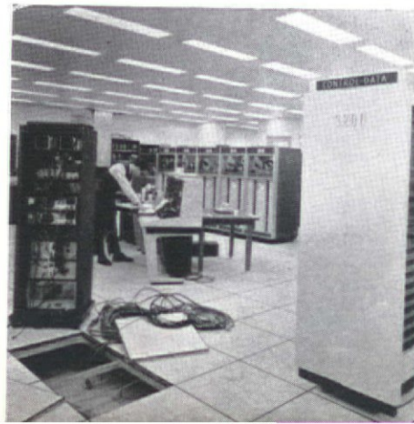
Liskey aluminum floor panels are lifted out to permit wiring at NASA's new computer installation (below left). Liskey's Elafloor is shown at IBM Data Center, Philadelphia (below right). Liskey also supplies special computer room partitions for such installations. Circle No. 166.
