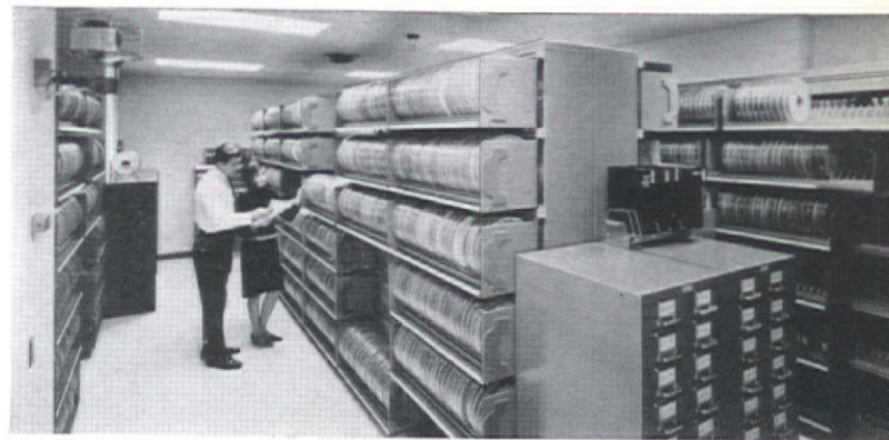
Tape vault in the new computer room of Prudential Insurance Co.'s corporate home offices in Newark, N.J. (above) uses Supreme's Conserv-A-File V. The space-saving unit has outer cradles that roll laterally to provide access to inner storage racks for fast tape selection. Circle No. 153.
