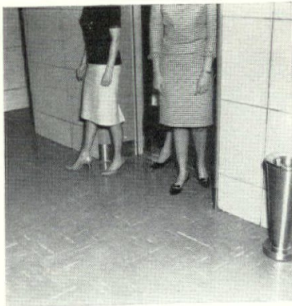
Wear tests at United Fuel Gas Co. were made in such heavy traffic areas as in cafeteria (right) and in elevator lobby (above). Estimating the life of vinyl asbestos tile, based on these studies, to be 25-30 years, United Fuel specified the floor covering for more than 50 branch offices.
