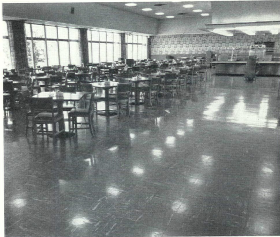
Wear tests at United Fuel Gas Co. were made in such heavy traffic areas as in cafeteria (right) and in elevator lobby (above). Estimating the life of vinyl asbestos tile, based on these studies, to be 25-30 years, United Fuel specified the floor covering for more than 50 branch offices.
