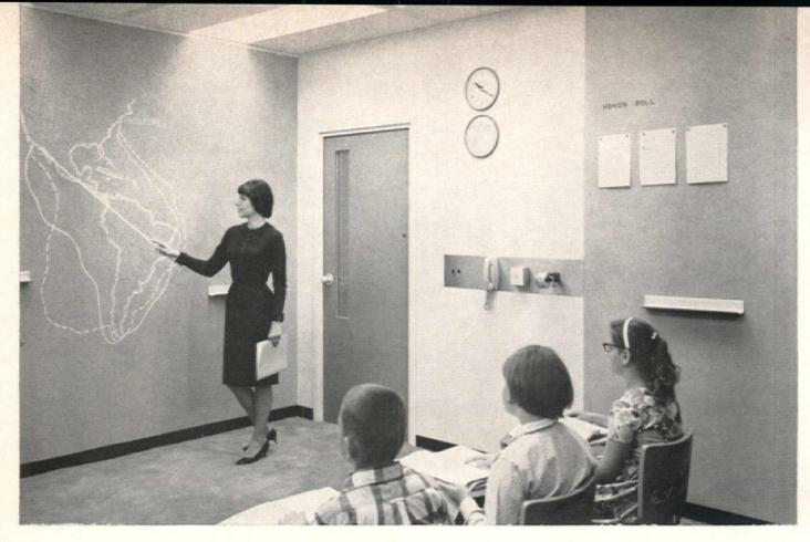
Hauserman's movable component classroom partition system has demountable double-wall chalk panels (at left) and service panels, fitted with clock, telephone, light controls. Its sound-retardant properties adds to its flexibility to meet all schoolroom requirements. Circle No. 104.
