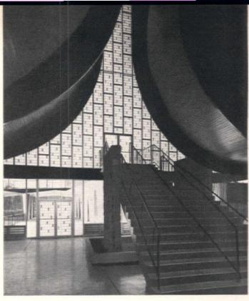
Panelux curtain walls, in a wide variety of patterns, grid variations, and colors, have acrylic modified polyester facing permanently bonded to a lightweight, treated cellulose fiber board core. The translucent sandwich panel is by Glidden Co. Circle No. 115.
