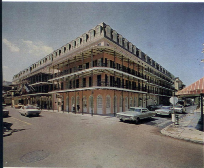
Downtowner Du Vieux Carre, a 186-room luxury motel-hotel located in the heart of New Orleans' French Quarter, is a showcase of that colorful city. As such, it demands a carpet that captures the charm and vitality of the city—Cabin Crafts. Every room in the Downtowner is luxurious from the floor up.
