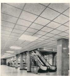
**CELOTEX CORP.**: Installation of Texture-Tone suspended ceiling gives an immediate face-lift to lobby of Central National Bank Building in Chicago. The larger, boldly fissured tiles are set in a grid system that integrates light and ventilation. Circle No. 104.
