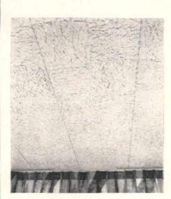
ELOF HANSSON: A popular and economical acoustical ceiling tile (above) is a deeply fissured, stone textured unit at close range, yet extends in a continuous visual flow at a distance. Circle No. 111. E. F. HAUSERMAN: A new textured metal pan system (right) has an overall sculptured appearance since the joints are virtually invisible. Sound is trapped as it passes through the plenum as well as through the material itself. Circle No. 112.
