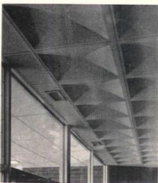
SIMPSON TIMBER: Suspended acoustical ceiling panels are outlined by exposed redwood grid runners in a reception area (far left). Circle No. 110.
