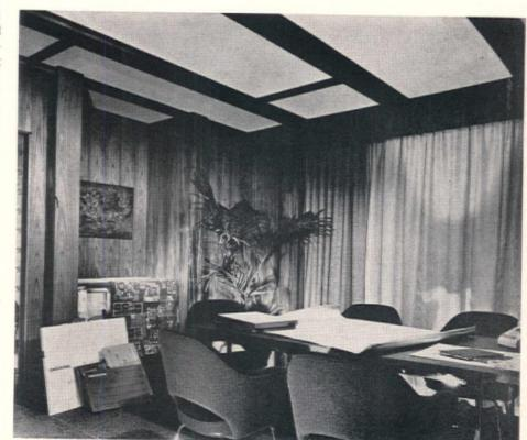
**OWENS-CORNING FIBERGLAS CORP.**: Architect's conference room is equipped with boxed beams that contrast with nubby texture of cloth-faced acoustical ceiling boards. Fiberglas ceiling is fire proof, available in any rectangular size, and can be installed in early building stages since the material is unaffected by humidity and temperature. Circle No. 108.
