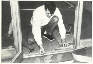
Combination of high break strength and low extensibility of jute backing was found to assure a permanently firm carpet installation, even after years of wear.
