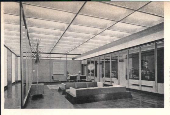
ARMSTRONG CORK CO.: New Luminaire suspended ceiling system combines high efficiency lighting, conditioned air delivery through tiny perforations in the panels, acoustical control, and fire protection in one integrated assembly. In addition, the exposed grid runner provides a positive connection from the ceiling to all partitions. Circle No. 101.
