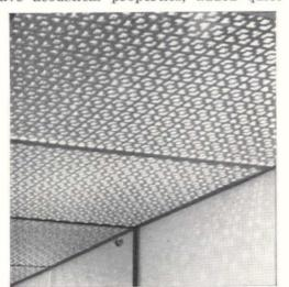
attained by providing the ceiling grilles with berglas blankets. Fire-resistant coating of the llework comes in a smooth white finish, which h be cleaned easily, or which can be painted. nels are available in 2 by 4 foot modules.
