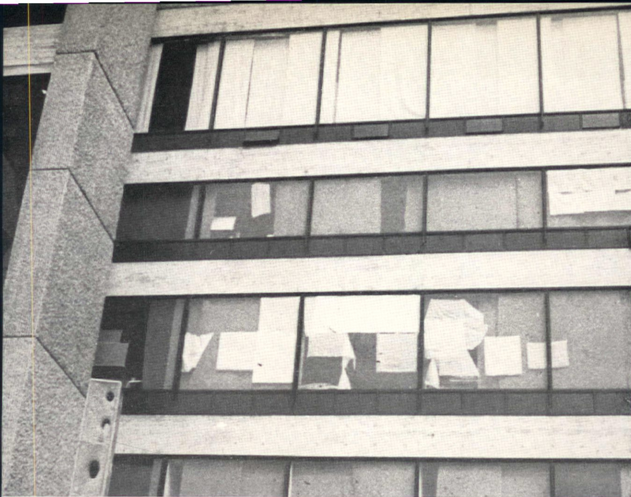
EXPANSES of glass (above) at Yale's School of Art & Architecture have made it difficult for students to work at their drafting tables in glaring sunlight. To cope with the problem, students have tacked up their work on windows, achieving "diffusion and reference" simultaneously, according to Mr. Lerner. Students on top floor, a neater group, used long sheets of fabric to cover continuous fenestration.
