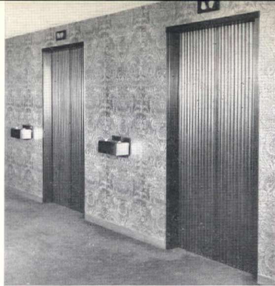
JAMES SEEMAN STUDIOS created an original wallcovering that is used throughout the Americana Hotel in New York City. Shown here installed in a corridor (left) and elevator area (above), the original design is a high-pressure laminate mounted on Pionite panels. Called Contessa, it represents a gold-on-white pattern silk screened by a special process.
