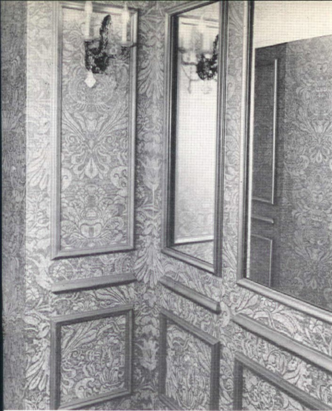
JAMES SEEMAN STUDIOS created an original wallcovering that is used throughout the Americana Hotel in New York City. Shown here installed in a corridor (left) and elevator area (above), the original design is a high-pressure laminate mounted on Pionite panels. Called Contessa, it represents a gold-on-white pattern silk screened by a special process.
