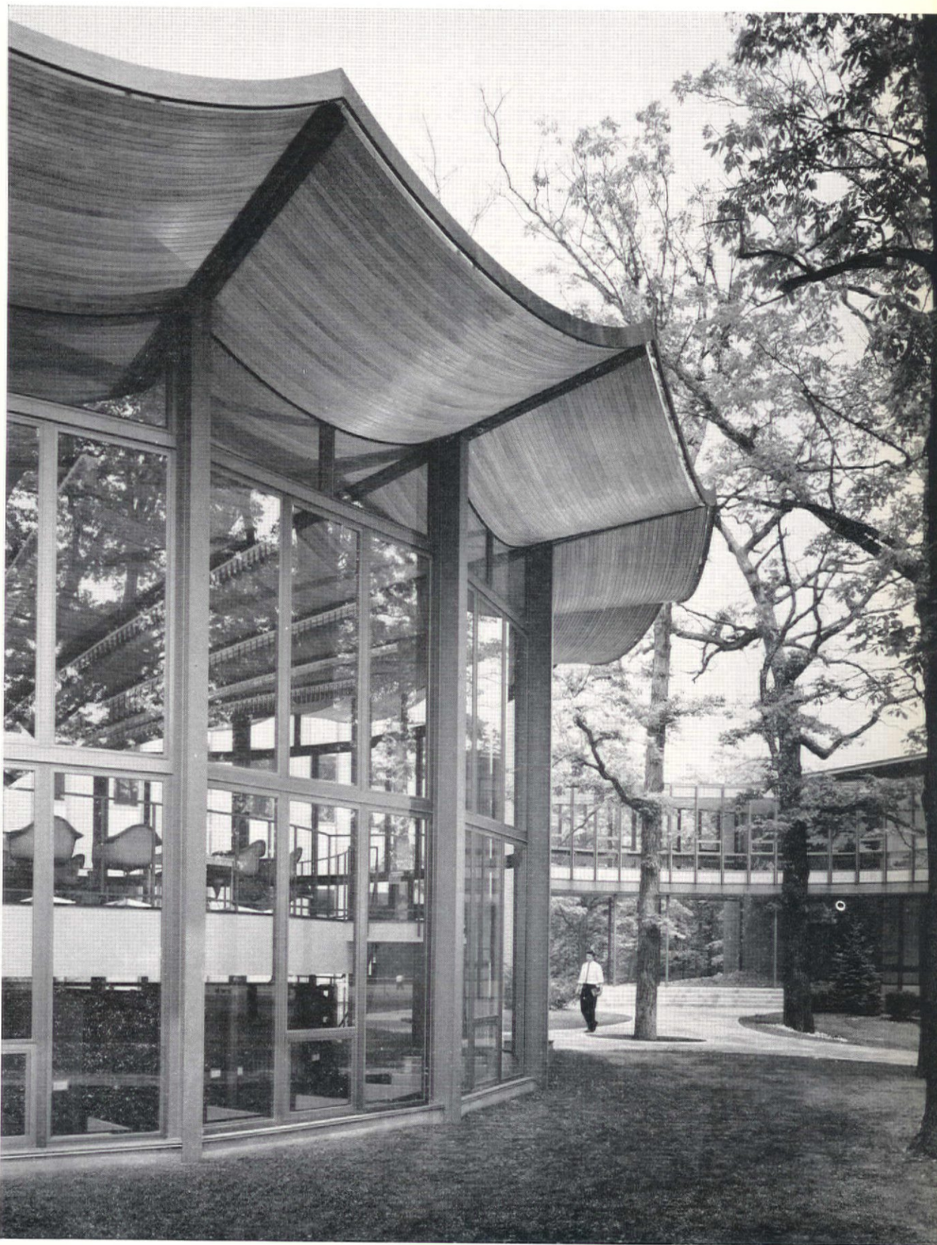
CIRCULAR science library at Lake Forest College, Lake Forest, Ill., by Perkins & Will, architects.
