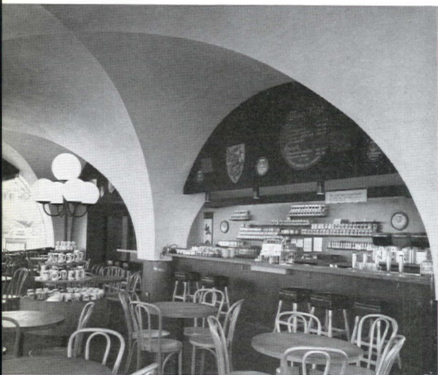
HOFBRAU HOUSE in Seattle's World's Fair is a low-cost contemporary vault structure, reminiscent of Bavarian Rathskellers. Building is bolted together and can be moved.
