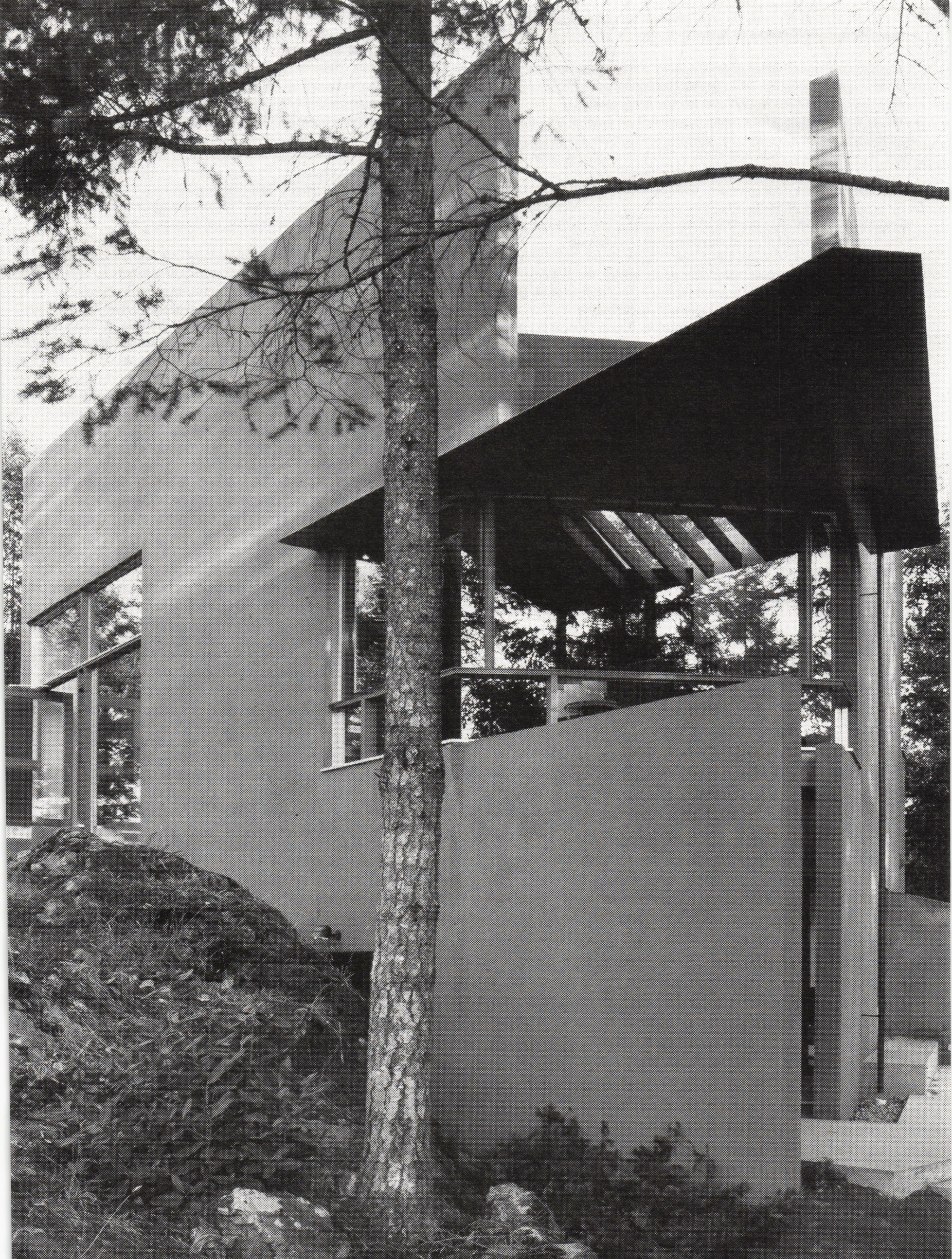
Barnes House: Nanaimo, British Columbia, 1991-93. Client: David and Fran Barnes. Architect: Patkau Architects. Project team: Tim Newton, John Patkau, Patricia Patkau, David Shone, Tom Robertson.
