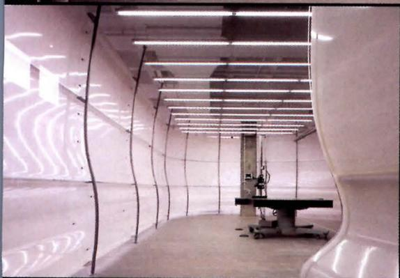
The cocoon panels (above and left) have flanges that fit into brackets welded to the curvy steel poles rising from floor to ceiling.
