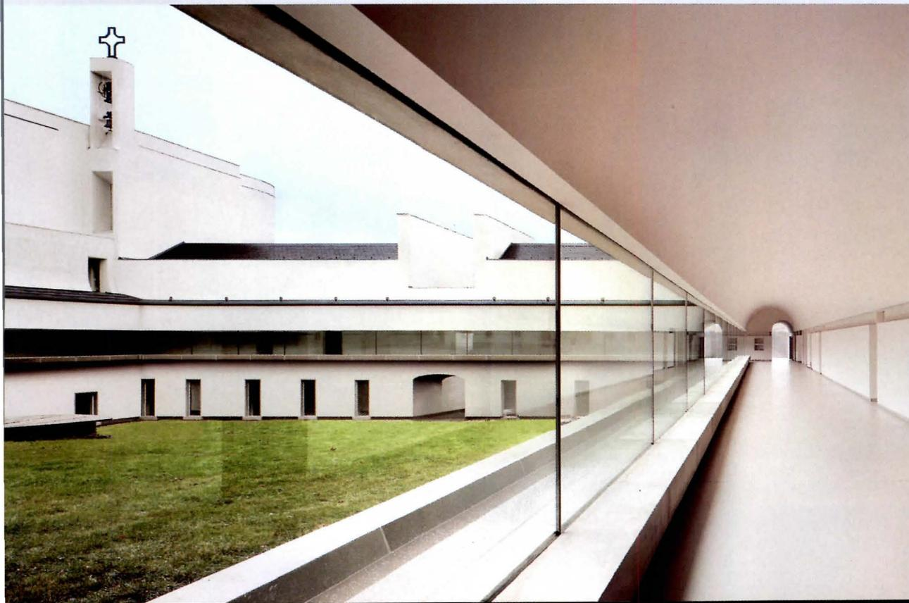
The ceiling of Novy Dvur's barrel-vaulted and glazed cloister cantilevers toward the grassy inner court, appearing to float over the slightly reflective resin-coated concrete floor. A continuous bench at the cloister's perimeter transforms into a rainwater trough on the exterior.
