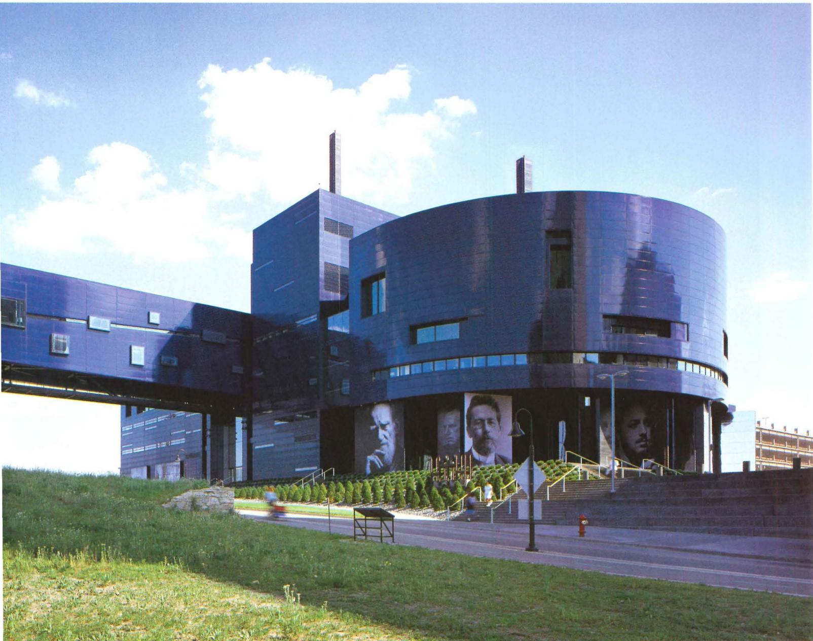
The zipper signs, visible from afar (right), evoke smokestacks, a sly reference to the “industry” of culture. The apsidal form (below) conforms to the shape of the thrust hall within. Patrons enter under a bridge that connects to set shops before proceeding to the lobby, located on the fourth floor.
