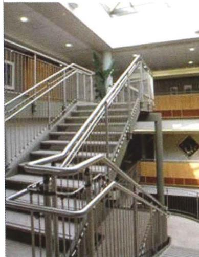
P & P Artec Modesto system, has 1 single round baluster. All fittings are powder coated. Their other systems include the Chicago – ( flat bar baluster). Double Baluster – (2 round balusters), and Munich – (3 oval baluster). Artec has built a reputation in 100% seamless handrail tubes. All of their systems are assembled and finished in the field, to provide each project a unique custom installation, without any visible joints.
