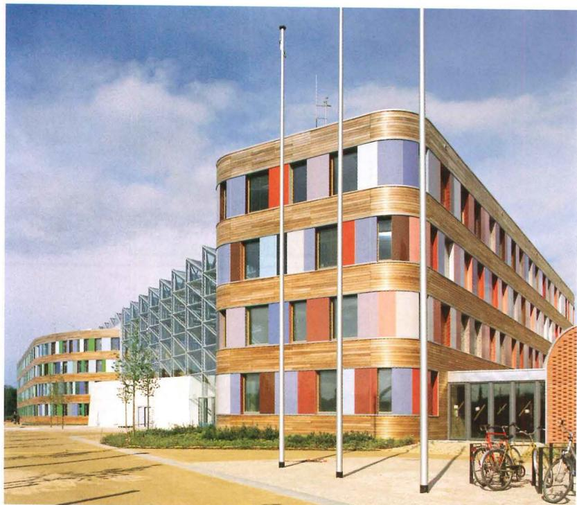
Daylight is admitted to the landscaped atrium through the serrated-glass roof (right). The offices in the double-loaded looping plan receive daylight and air through use of operable windows. All employees have their own offices with windows, and ones overlooking the atrium seem to be favored.
