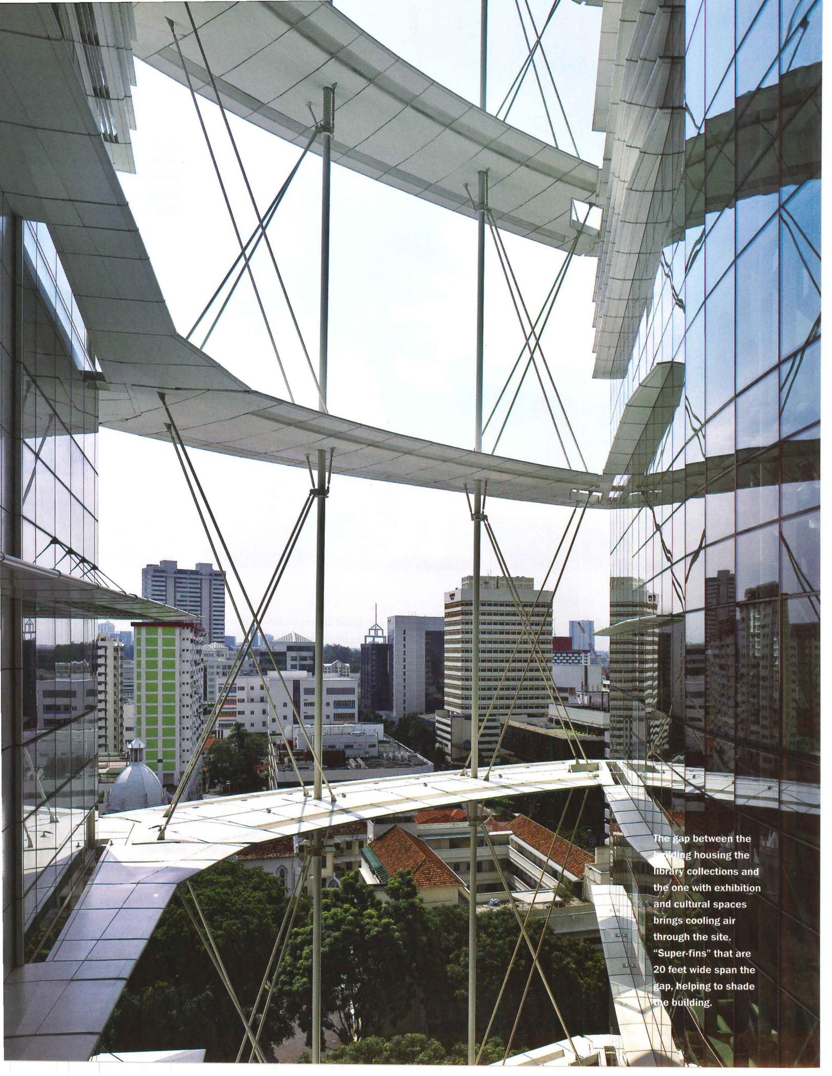
The gap between the building housing the library collections and the one with exhibition and cultural spaces brings cooling air through the site. "Super-fins" that are 20 feet wide span the gap, helping to shade the building.
