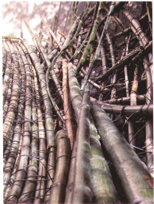
**The bridge, made from approximately 150 locally harvested bamboo shoots and connected with 2,000 cable zip ties, can be seen from the street, inviting passersby to enter this experimental space and interact with the entire installation.**
