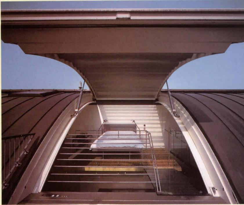
The operable skylight of this London apartment by Brookes Stacey Randall (left) is made of aluminum to reduce the load on the hydraulic openers. The section was manufactured off-site and lifted into place by a crane (far left).
