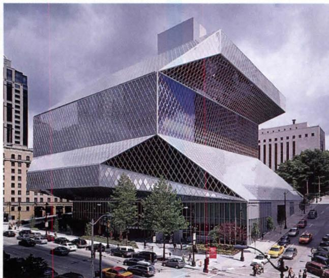
Projecting forms (supported by enormous cantilevered trusses reach for views. The steeply sloping site—two floors in a city block (opposite)—adds to the kinetic effect. Fourth Avenue entrance (near left) opens to children's area. The gridded curtain wall peels away to form arcade at the main, Fifth Avenue entrance (far left and below).
