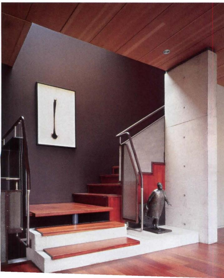
material palette of concrete and painted steel that play against polished mahogany floors and Douglas fir ceilings. There's a strong nautical influence in the painted steel columns, curving handrails, and slatted-wood ceiling above the entry hall and the stepped walkway down to the lap pool. Inspiration also comes from Alvar Aalto, traditional Japanese wood construction, and the borderline-obsessive detailing of Carlo Scarpa, a frequent reference for Shim and Sutcliffe.
