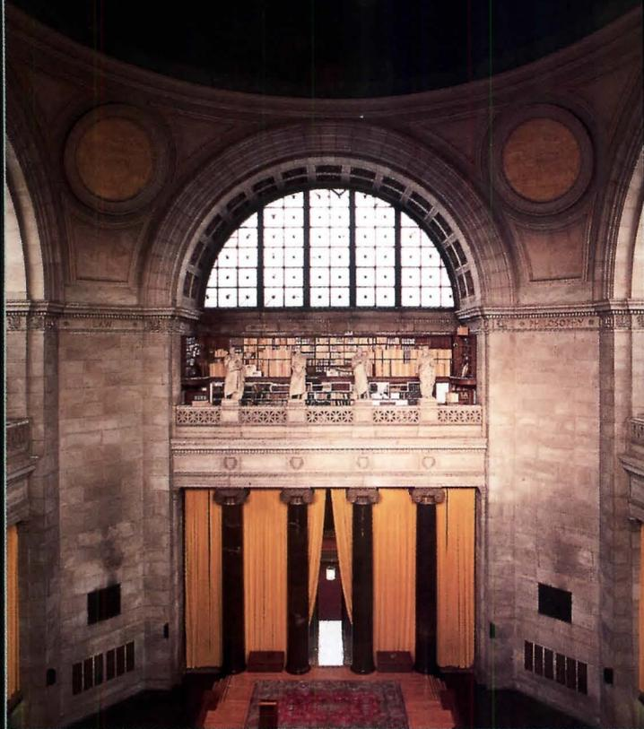
The monumental stone arches visible inside the rotunda only do a small part of the job of supporting Low's masonry outer dome. Huge brick arches (right) built on top of the stone ones do the real work. These
