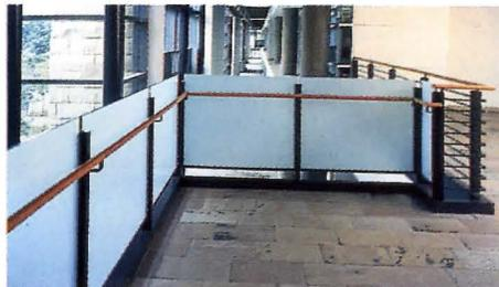
providing glass safety and UV-protection, the films now offer a wide range of colors, patterns, designs, and textures, including frosted white, opaque (shown), square and striped designs, and small and large dots. Many
