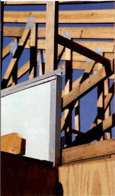
conforming to the requirements established by the representative fire test and the manufacturer of the area separation wall system. Use of a noncompliant clip, or elimination of the clips altogether, may result in the failure of the system to work as intended.
