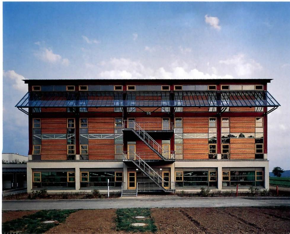
With the lines between factory and office blurring, it's only natural that techniques useful for offices can also be applied in a manufacturing setting. A case in point is this 36,000-sq-ft timber-framed production-hall addition to the campus of furniture maker Wilkhahn. Munich architect Thomas Herzog suspended wood and metal trusses for clear-span production spaces between trestle-like towers that contain
