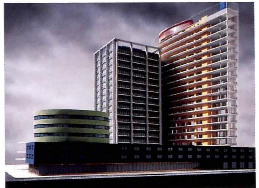
the facade and heat gain is less because mornings are cooler. The shutters are located within a 1m (39-in.)-wide thermal flue (a readily maintained size), which exhausts heat accumulated from the sun and from offices via the stack effect. The flue also draws fresh air from east to west. A wing-like roof structure creates an airfoil so that prevailing breezes augment the natural buoyancy of waste heat. Individ-
