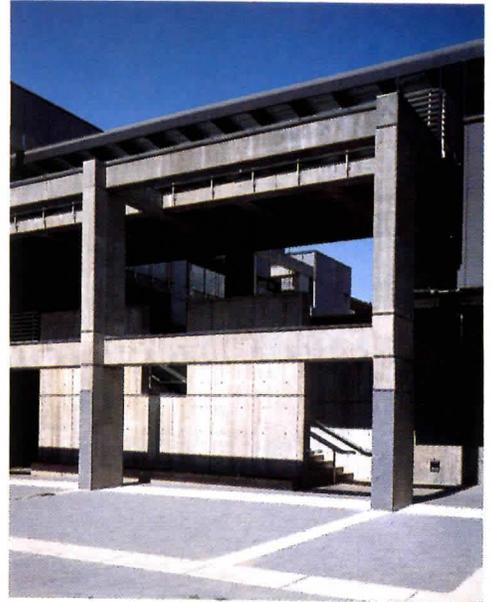
*Kieran Timberlake & Harris used smooth forms for concrete at the University Center at East Stroudsburg University (RECORD, October 1993, pages 110-111). Granite coping stones protect horizontal surfaces exposed to weather.*
