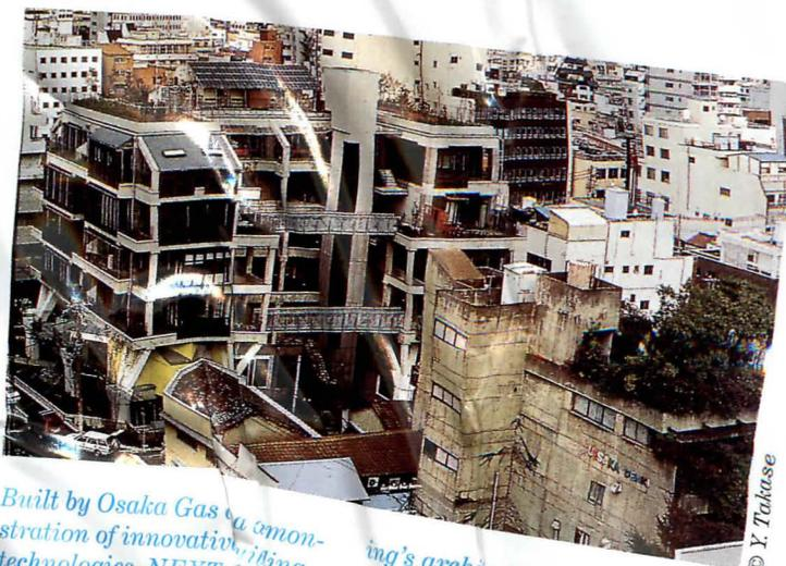
Built by Osaka Gas as a demonstration of innovative building technologies, NEXT21 employs an "open building" system as well as new approaches to reducing energy consumption and waste production.
