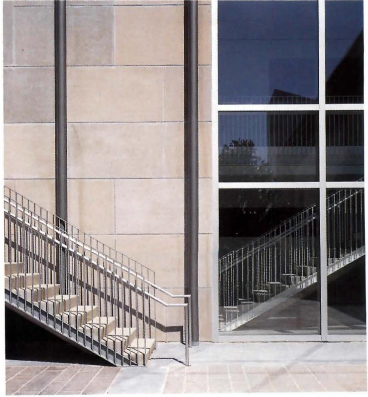
*Jimenez has foregone his typical palette of vivid colors for the subdued tones of limestone and clear anodized aluminum. The simple volumes are crisply detailed. Windows are either ganged together and held flush with the stone face or treated as singular, deeply punched openings.*
