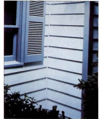
InnerSeal<sup>®</sup> lap siding is made from small-diameter, noncontroversial trees and has exceptional moisture resistance to resist weathering, splitting or curling. Uniformly light in weight, they are unsurpassed in dimensional stability and durability. Siding is finished with a protective overlay that's pre-primed to hold paint and stain longer. The look of solid sawn siding without the expense, the waste, or the work.
