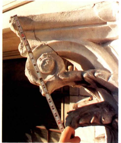
2. This crack was filled with sealant. The stone should have been repaired by injection of a bonding agent (sealants' adhesive bond with stone usually fails shortly after installation). Better yet, it should have been replaced.
