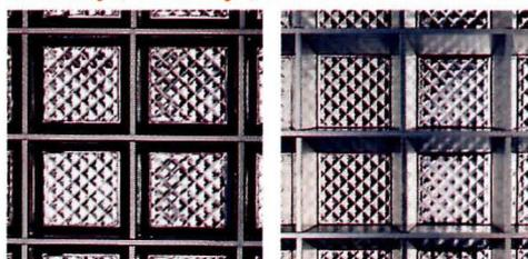
Horizontal panels employing IBP's mortarless, brushed aluminum, modular frame system and PC GlassBlock® paver units are equally attractive from above or below. Walkways, up to 72" wide, in any length, meet code requirements for supporting specific loads.
