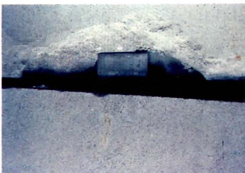
Ignoring stresses at clip angles, especially from movement of adjacent panels, can lead to spalling (above).
