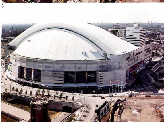
which framing would be left behind when the roof was opened (the shadows cast would reduce television-signal quality). On the other hand, the competition brief required that the retracted roof remain within the site's tight property lines. The final scheme combined aspects of what Robbie and Allen call the grapefruit analogy—rotating wedges—and telescoping parabolic vaults. The solution leaves only the northernmost nine percent of the stadium (beyond center field) under fixed cover.
