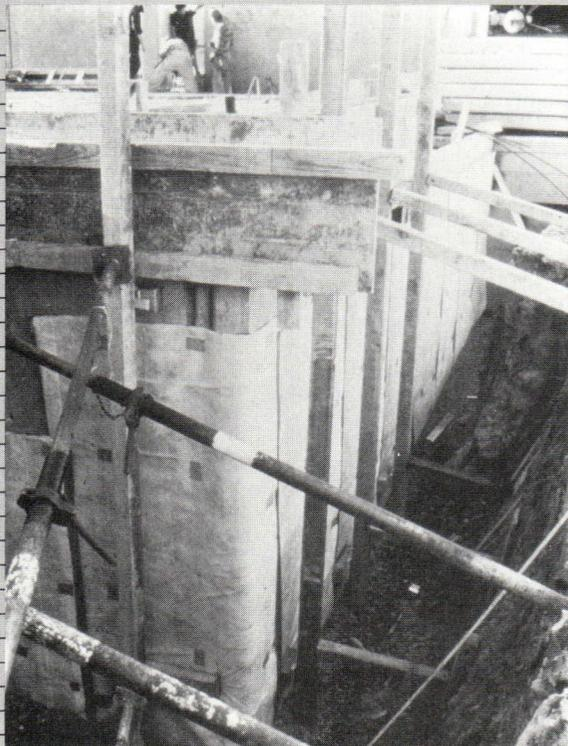
Armco STRIPDRAIN 75 drains more water than a 14'-thick sand or 17"-thick gravel drain.
