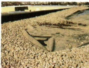
distributes stresses caused by wind uplift. The non-penetrating attachment in fig. 6 shows the membrane movement caused by the wind, which can result in seam failure (fig. 4). Wind uplift can also redistribute ballast (fig. 5), leading to roof failure.
