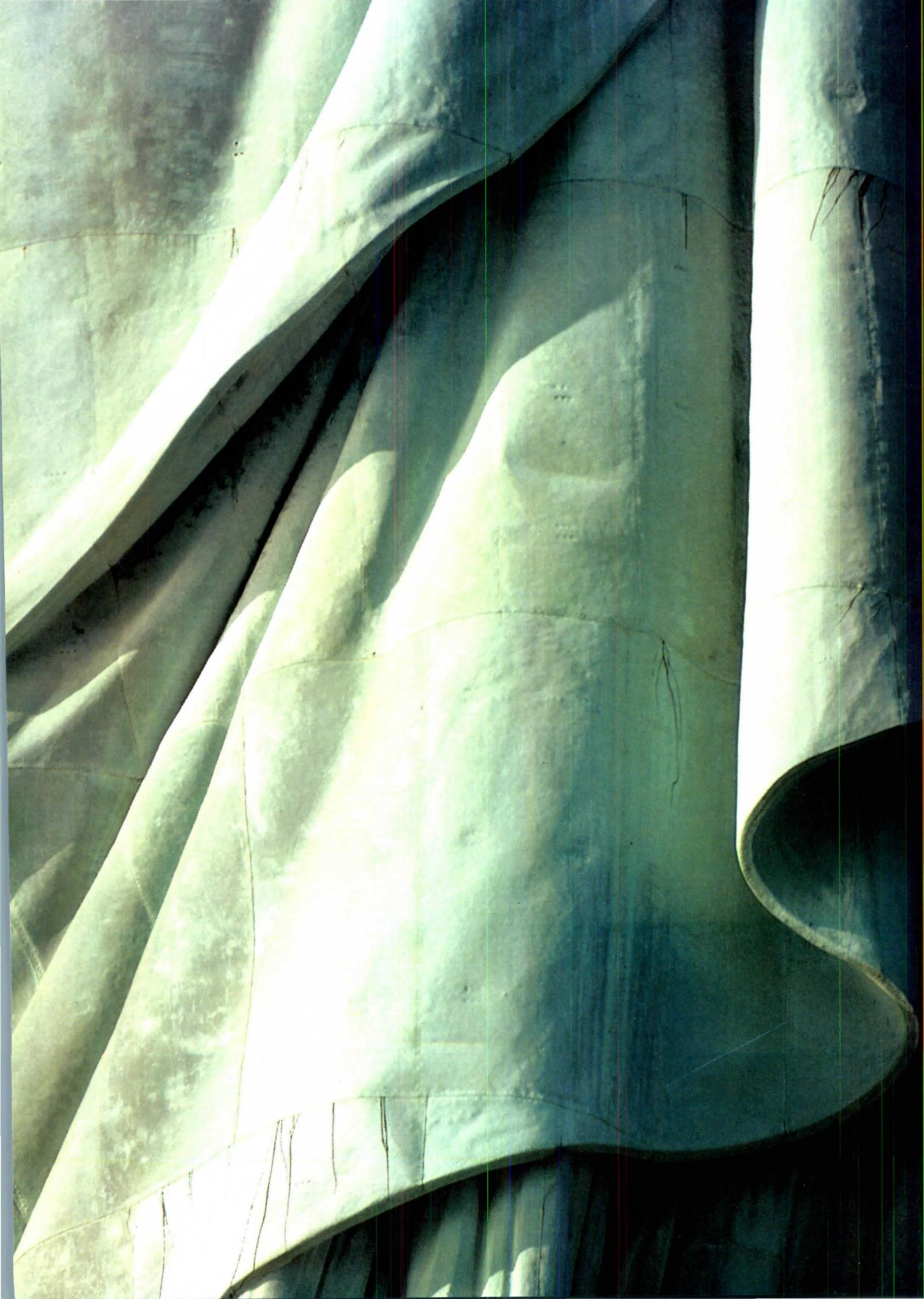
While the outer copper skin of the Statue of Liberty has few damages visible to the naked eye, the scaffolding that now veils the entire statue will be used for closer looks and chemical tests. Coal-tar leaks at the seams will be cleaned and dents hammered out, but basically the skin will remain as is: the verdigris has both esthetic and technical value—the oxidation provides a chemical shield.
