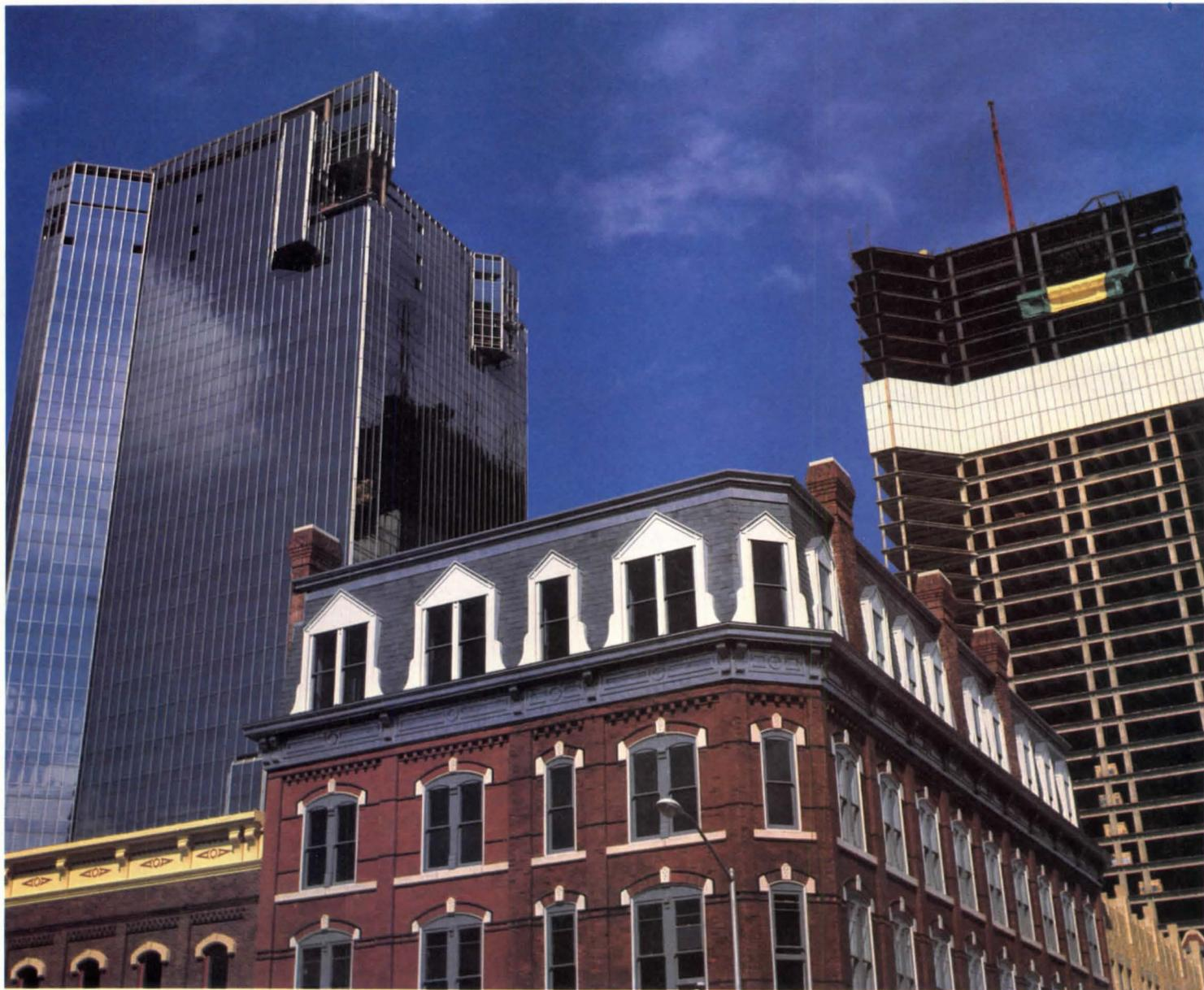
*Exposed tripod and clustered-pair columns are scale-relating elements for Tower 1 (left) and Tower 2 (right) in City Center, which also embraces two blocks of historic building renovation (foreground) by the same developer. Rudolph expressed the plasticity of the curtain wall with turrets at top and bottom and wings at corners, and he notched Tower 1 to admit daylight to a skylight.*
