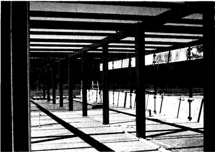
truss, combined with floor and ceiling beams and with cladding for exposed units. For this hospital construction, the same 3.6-meter grid was used for both the two- and three-bay units. The structural floor consisted of light steel beams and a steel plate diaphragm, while 4-in. precast concrete panels with an exposed aggregate finish were used for the exterior skin. Also included in each module were plumbing, hvac and electrical systems designed with special connections at the module joints.
