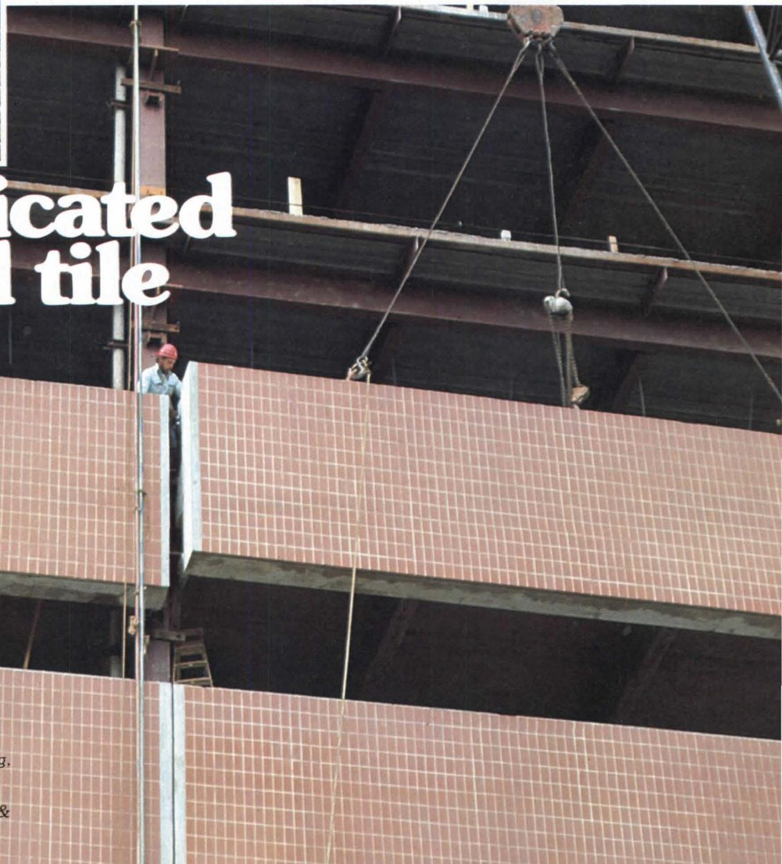
Harristown Key Block, Phase 1, Harrisburg, Pennsylvania. Over 240,000 sq. ft. of Gail tiles set in precast tile panels, 8'8" x 30 ft. Architecture: joint-venture, Lawrie & Green - Mitchell / Giurgola.
