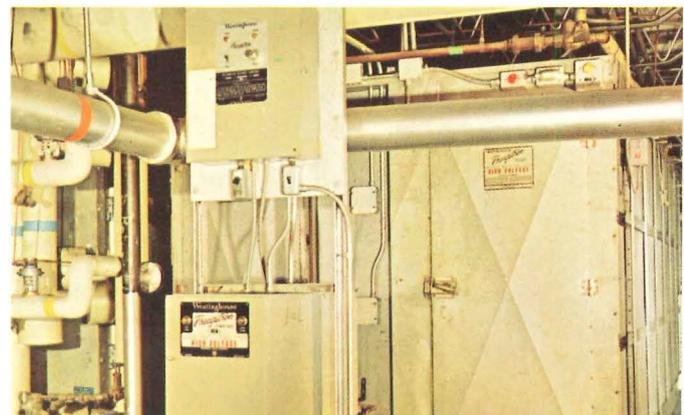
D. Westinghouse Precipitron® electronic air cleaner removes up to 95% of all dirt particles, smoke and pollen circulating throughout a building. Traps particles as small as 1/100th micron. Holds contaminants on electrically charged plates, without reducing flow of air through the cleaner.
