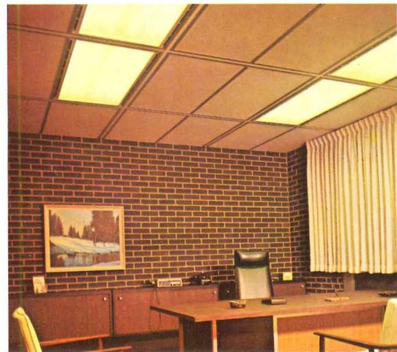
P. Westinghouse space-saving ceiling system gives lighting, acoustical control and air handling capability in one installation. Flexible to fill individual requirements. Eliminates separate lighting and air-handling fixtures. Gives architect complete design freedom.
