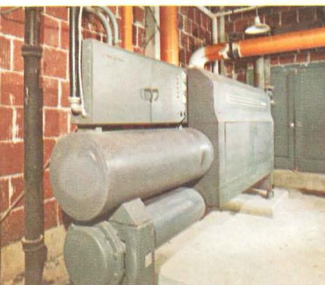
F. This 137-ton PE direct expansion packaged chiller fits through a 30-inch door. Installed in three-story addition to the Sheffield Memorial Building, Atlanta, Ga., it is completely factory assembled, pretested and charged. Also included in job are Westinghouse-Sturtevant fans and air handling equipment.
