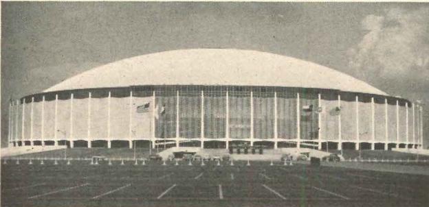
Take a circle, cap it with a dome, and you may have the makings of an acoustical horror. Uncontrollable reverberation or "bounce" produces echoes which in turn cause ear-splitting feedback throughout the sound system. Add to this up to 66,000 cheering Texans who want to hear as well as be heard and you have a sound problem seeking a solution.
