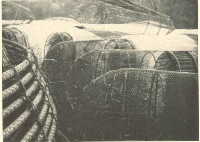
Where vaults abutted the compression-tension ring, the lath was given a double-curvature shape similar to a fencer's mask.
