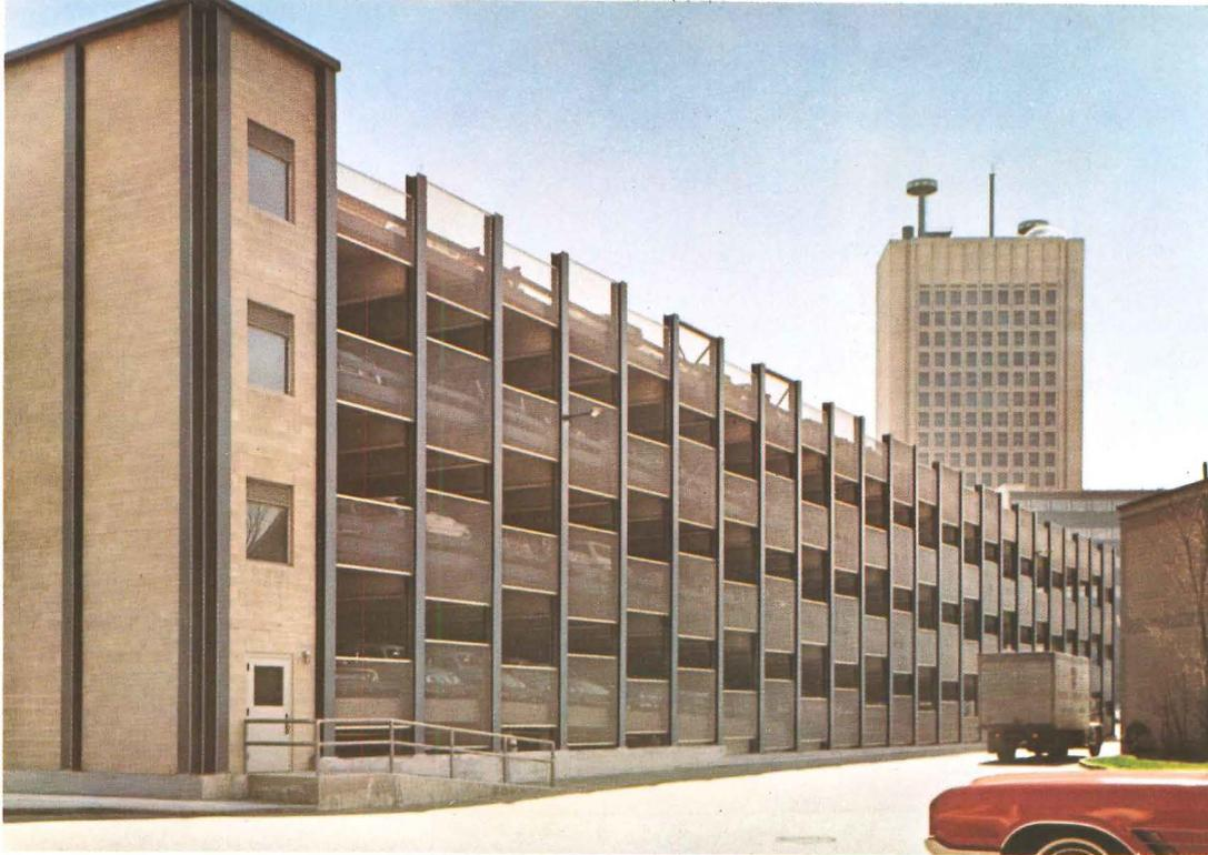
**Skillful execution of exposed structural steel framing** is the key element in the design of the M.I.T. Parking Facility—No. 1, East. Basic structure is a rectangle, 228 ft x 121 ft, within which 425 standard-size cars can be parked on each side of 60-ft-wide inclined ramps. Main parking areas are column-free to make maximum use of space. Mesh enclosure panels between the exterior columns serve as snow fencing and enhance the structure's appearance.
