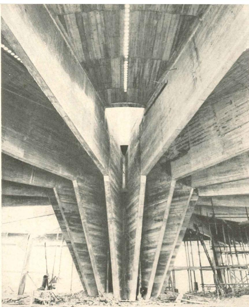
Variations in the tone of the concrete fins at the base of the water tower, Caen La-Gueriniere, France, result from casting against formwork made up of boards with different degrees of absorbency, and from bleeding at joints.
