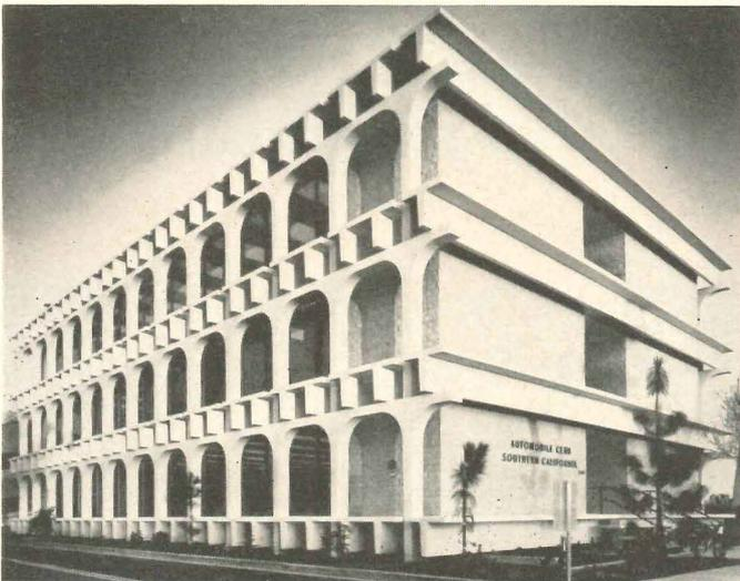
"A pure expression of all structural elements and their functioning both on the exterior and on the interior. Prestressed concrete single tees and tree forms, as well as long span elements, are carefully correlated. They express themselves as an architecture of their own."
