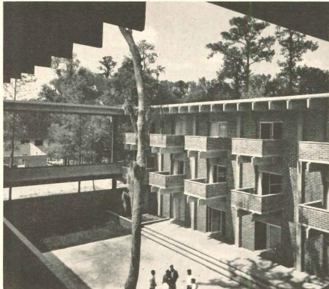
"A straightforward articulation of prestressed concrete units. It shows a variety in the play of light and shadow and in texture and surface not ordinarily associated with prefabricated component parts."
