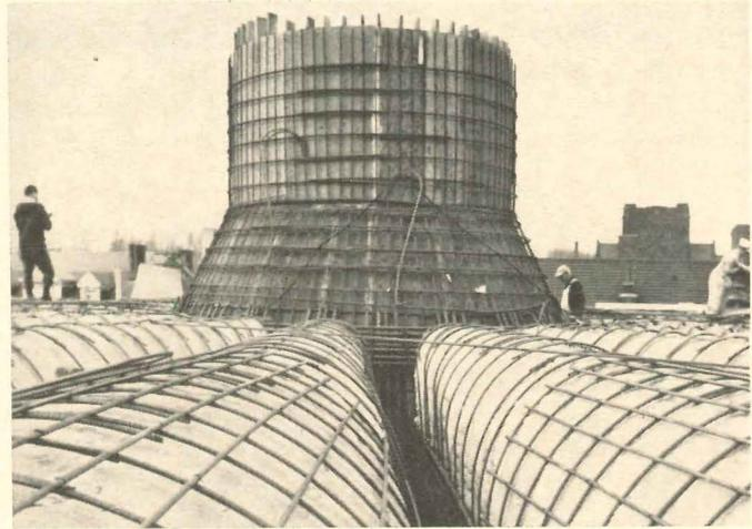
An integral tough skin on the top surface of the insulation allowed the placement of slab bolsters and reinforcement.
