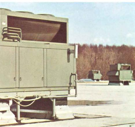
E. Zoned heating and cooling control is provided by ten Westinghouse IC Roof Mounted units at the Xerox Corporation's Eastern Regional Distribution Center, Blauvelt, N.Y. The unit's low silhouettes do not interfere with looks of building. Four capacities available: 7½, 10, 15 and 20 tons.
