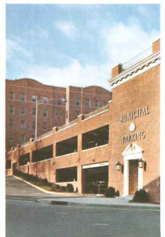
**Traditional for Mount Vernon, N.Y.** The cast-stone trim, wrought iron railings, and brick facade of this parking structure conform to the colonial character of surrounding municipal buildings. The two enclosed levels and exposed upper deck provide a 320-car capacity. Bethlehem V45 steel was used for the framework. This high-strength grade was a major factor in achieving an extremely low per-stall cost.
