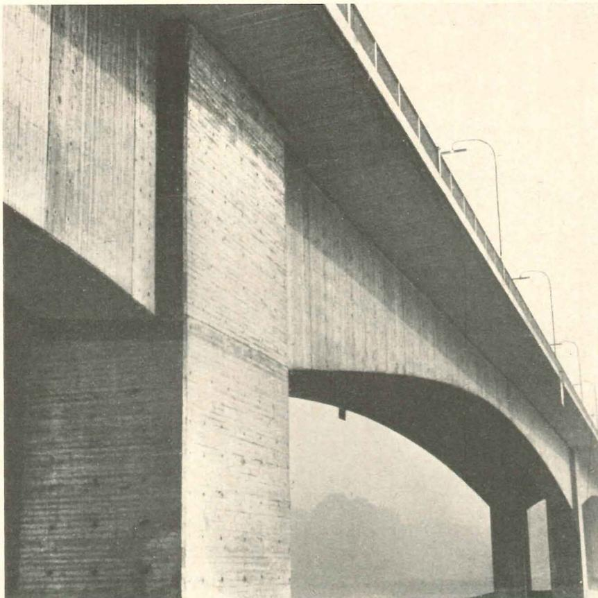
In order to preserve uniformity of color, new and used boards should not be part of the same formwork. The dark concrete area at the top-left-hand corner of this photograph is probably due to the use of a panel of new formwork.
