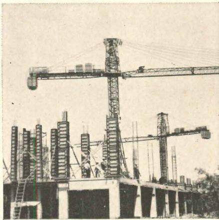
Using the Symons Slab Shore System for all floor slab forming, the concrete sub-contractor on the new Hague Towers luxury apartments in Norfolk, Virginia, completed each 15,500 sq. ft. floor in a 6-day period.
