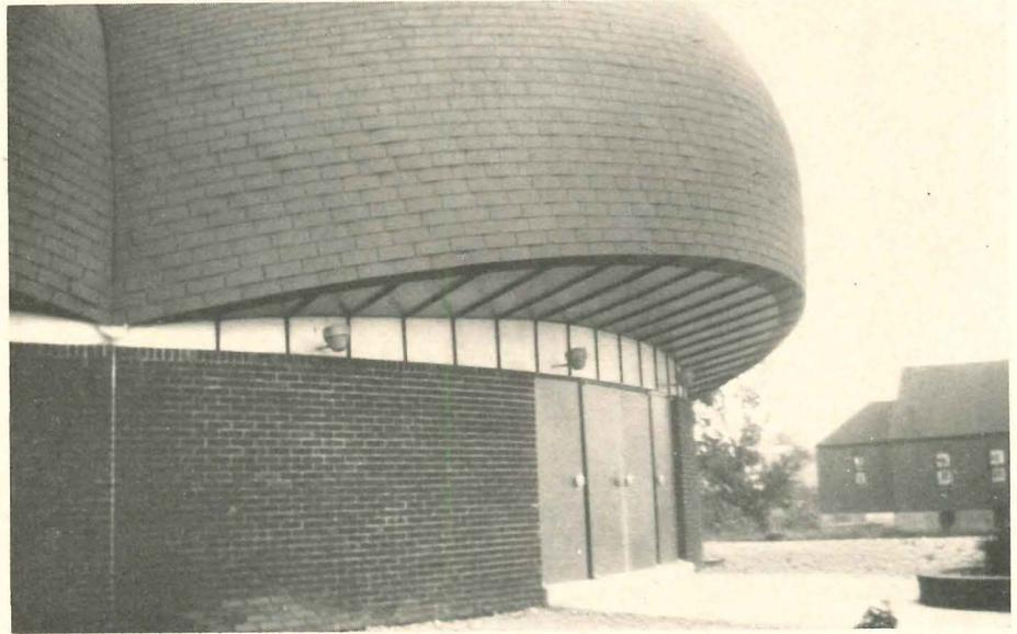
Most of the light, natural and electric, enters through wired glass panels.
