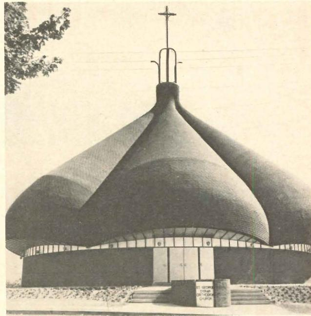
panels. The top of the 7 ft 8 in. wall, directly below the glass panels, consists of sand-float finish, white stucco, based on metal lath in order to follow the circular form of the foundation of the church. The ground at the foot of this wall is covered with a bed of white river stone. The vertical white panels and the bed of white river stone reflect natural light upward, through the glass panels to the curved ceiling of the church.
