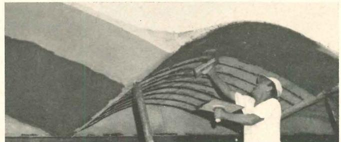
Applying brown coat of plaster to underside of the canopy.
