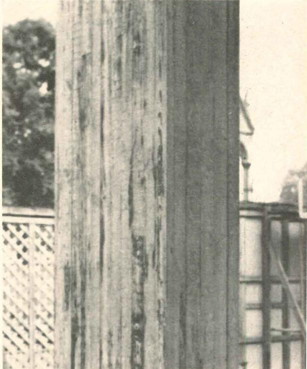
Formwork made up of low grade timber cut from various parts of the trunk or at different angles through the sap channels varies widely in absorbency and results in substantial color variation in the concrete finish.
