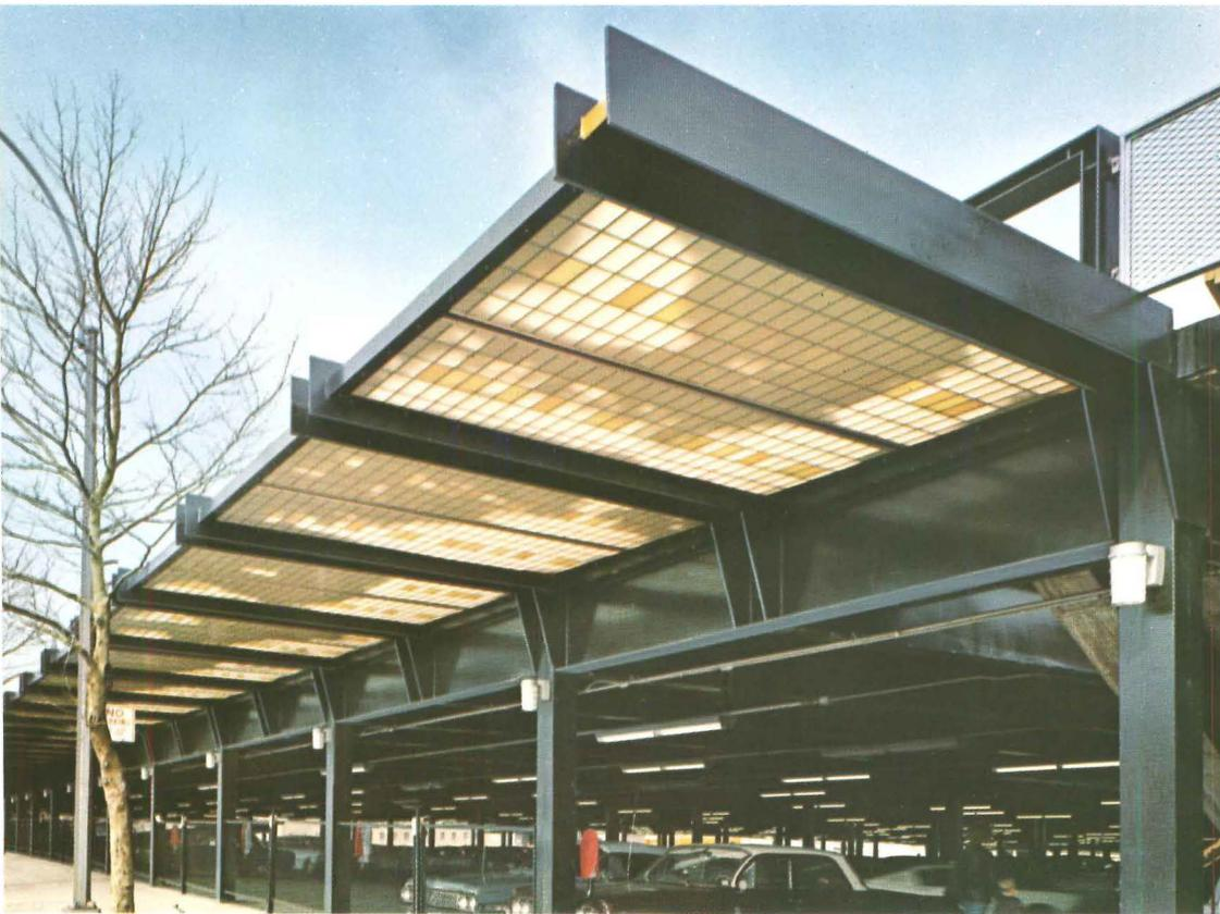
**New deck over existing parking field.** It's the Municipal Parking Field in Flushing, N.Y.C. Capacity: 1,130 cars. All structural components are at 8 ft, 6 in. centers; columns are spaced at 62 ft on centers. Main outrigger supports for plastic shelter canopies are 12-in. WF with web horizontal to harmonize with the stepped railings. The New York City Department of Traffic is so pleased with its appearance—and its low cost—that they are planning another structure of similar design.
