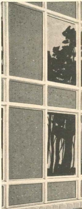
**1. PRE-CAST CONCRETE PANELS.** Problem: Water leakage around pre-cast concrete panels in curtain wall and tilt-up construction. Solution: DAP Flexiseal. Conforms to all irregular sealing surfaces, makes a tough bond for watertight, airtight protection. Gives long-term, trouble-free service.
