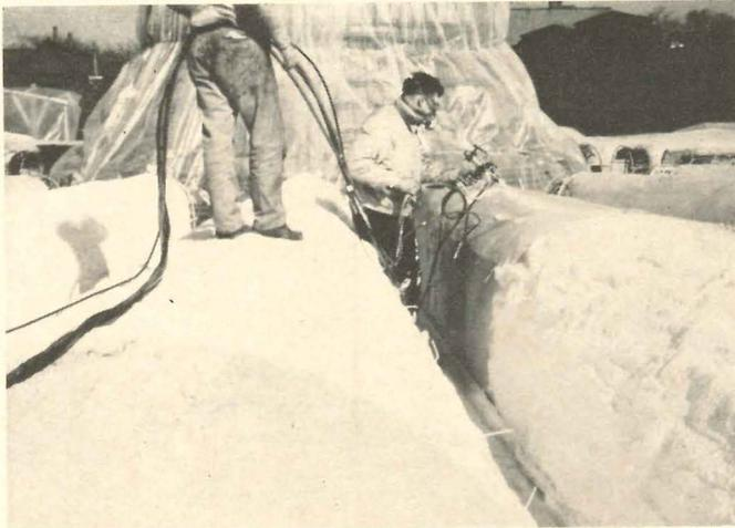
Polyurethane insulation was sprayed onto the plaster surface. It grew in thickness from approximately  $\frac{1}{8}$  in. to  $1\frac{1}{4}$  in.
