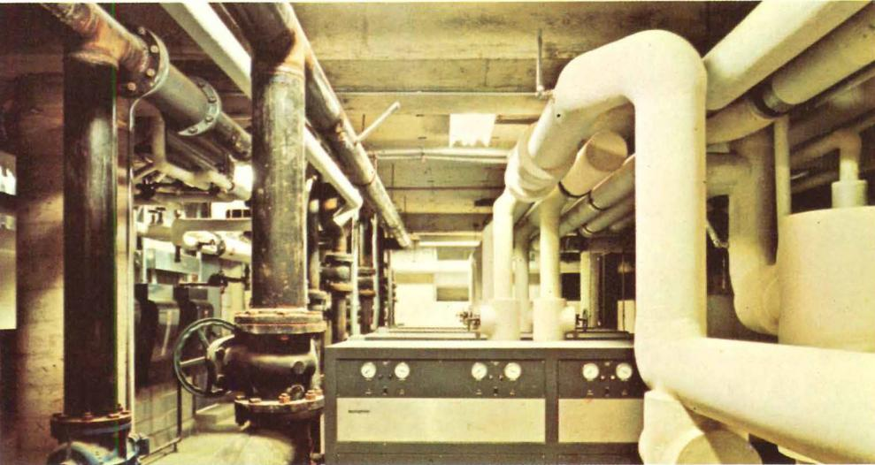
L. Four 60-ton packaged chillers air condition 250,000 sq. ft. of ballroom and adjoining banquet rooms in the Shoreham Hotel in Washington, D.C. Cooling controlled in 12 steps to suit various-sized crowds and outside temperatures. Quiet, reliable operation through factory pretesting, Guardistor® motor protection and single-unit construction.
