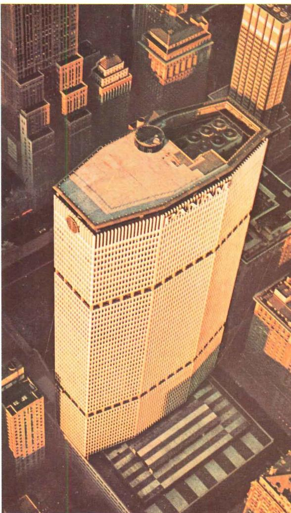
G. In the famous Pan Am Building, world's largest commercial building, every cubic inch of air is handled by Westinghouse equipment. Total of 82 Westinghouse fans includes Centriline® fans, industrial fans and centrifugal fans. 236 Westinghouse specially designed large air handling units complete the job.
