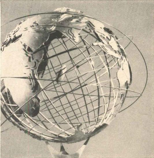
**UNISPHERE:** Symbol of the Fair, this "biggest world on earth" required wind tunnel studies and computer aid for efficient design. Wind loads were sizably increased by the concave inner surfaces of the large stainless steel land masses. Despite its lacy look, Unisphere is sufficiently stable to withstand a hurricane. Unisphere® presented by USS United States Steel © 1961 New York World's Fair 1964-1965 Corporation.
