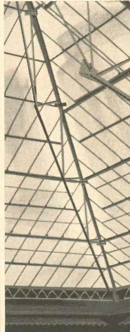
**5. SKYLIGHTS.** Problem: Temperature extremes and wind pressure cause excessive movement of glass lites with resulting breakdown of seal between glass and metal frames. Solution: DAP Flexiseal. Sticks tenaciously to glass and metal, flexes indefinitely to maintain positive, long-lasting seals.
