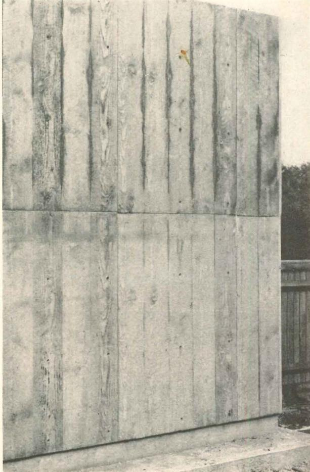
Hydration discoloration here is caused by loss of moisture at the board joints.
