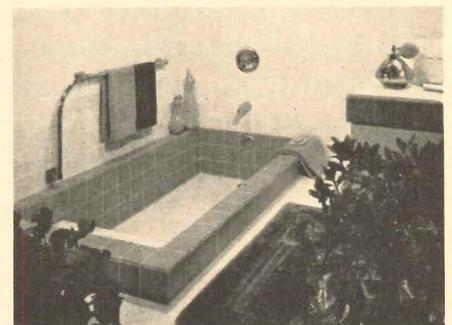
the rough framing. Special design of the tub permits second floor installation without a drop ceiling. When tiled with ceramic tile, and color coordinated with decorative wall tiles, conventional bathrooms acquire a sense of luxury. Tiles on the wall in the photo are one of Max Spivak's recent designs for the company. *Cambridge Tile Manufacturing Company, Cincinnati, Ohio*
