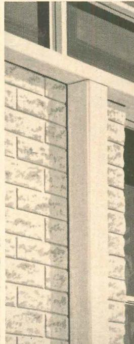
**4. EXPANSION JOINTS.** Problem: Shear stress causes adhesion or cohesion failure of ordinary sealants between dissimilar materials. Solution: DAP Flexiseal. Provides outstanding shear strength for tough, flexible, long-lasting seals between aluminum, brass, copper, steel, glass, concrete, marble, wood.
