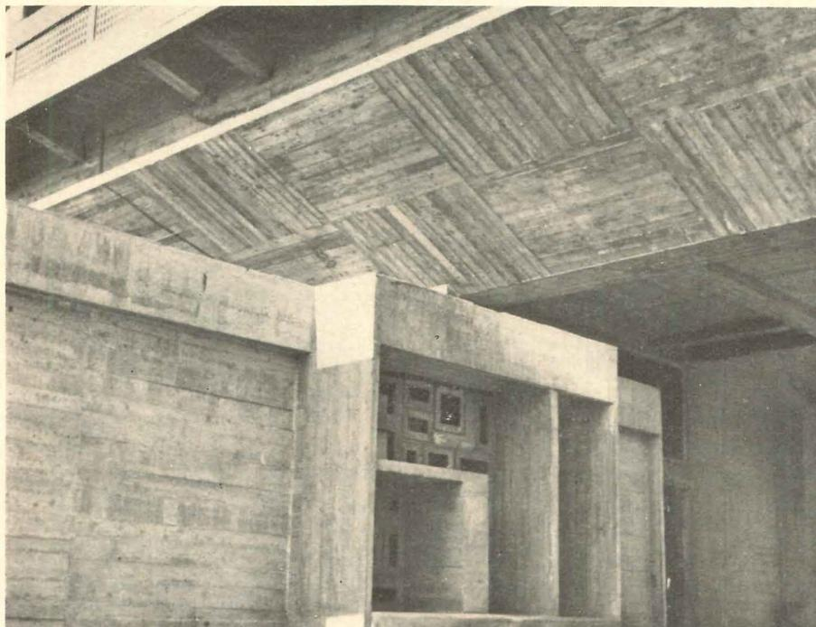
Technological imperfections and blemishes can be clearly seen in the entrance hall and board marked soffit of the first floor of the Unite d'Habitation, Marseilles. For Corbusier, however, these are an accepted part of his personal concrete esthetic.
