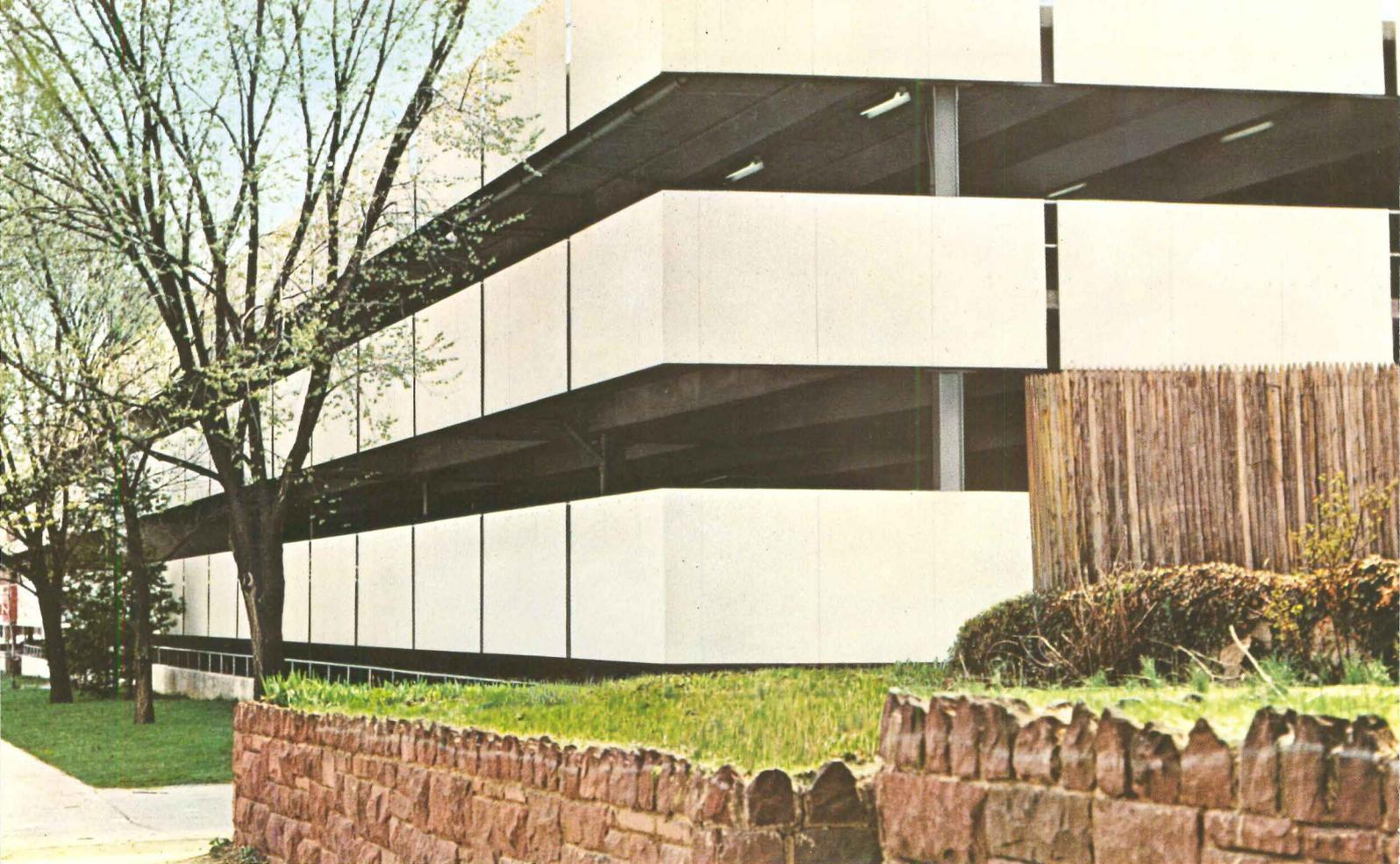
**Framed in steel for a light, floating appearance.** This four-level parking structure for a Sears Roebuck store in Washington, D.C. can accommodate 1,000 cars. Located in a residential neighborhood, its long, low silhouette blends nicely with its environs. The lightweight colored panels, which hide the cars from passersby, give the building a "finished" look seldom found in parking structures.
