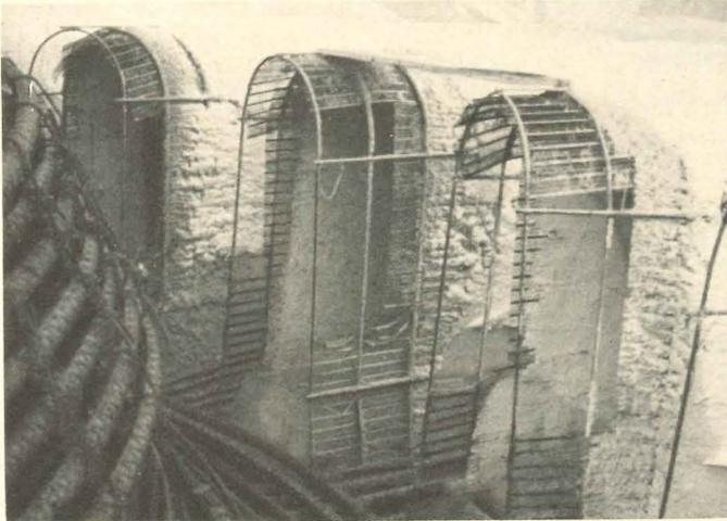
Arched ribs of reinforcing rods supported metal lath which was given a brown coat of plaster followed by insulation.
