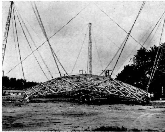
*The top ring of five triangles and the second ring are lifted 3 ft off the ground with ginpoles to permit addition of next ring*
