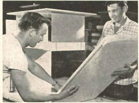
With refrigerating units installed, the cabinet is assembled to the back sheet. The steel doors are attached, and the unit is ready to be "built in" as shown
