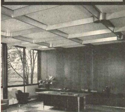
This executive office in the Research Administration Building, one of seven at the General Motors Technical Center air conditioned by Thermotank, shows a typical installation of Thermotank's custom-designed diffusers with integrated sprinkler heads
