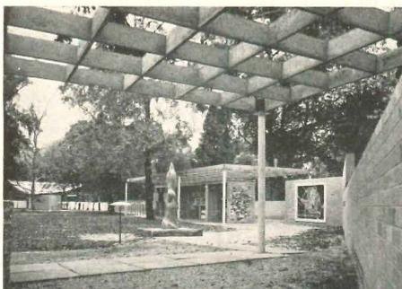
*pavilion (center) is composed of six bays of 18 ft span prestressed periphery beams which carry a 3 ft grid of post-stressed*
