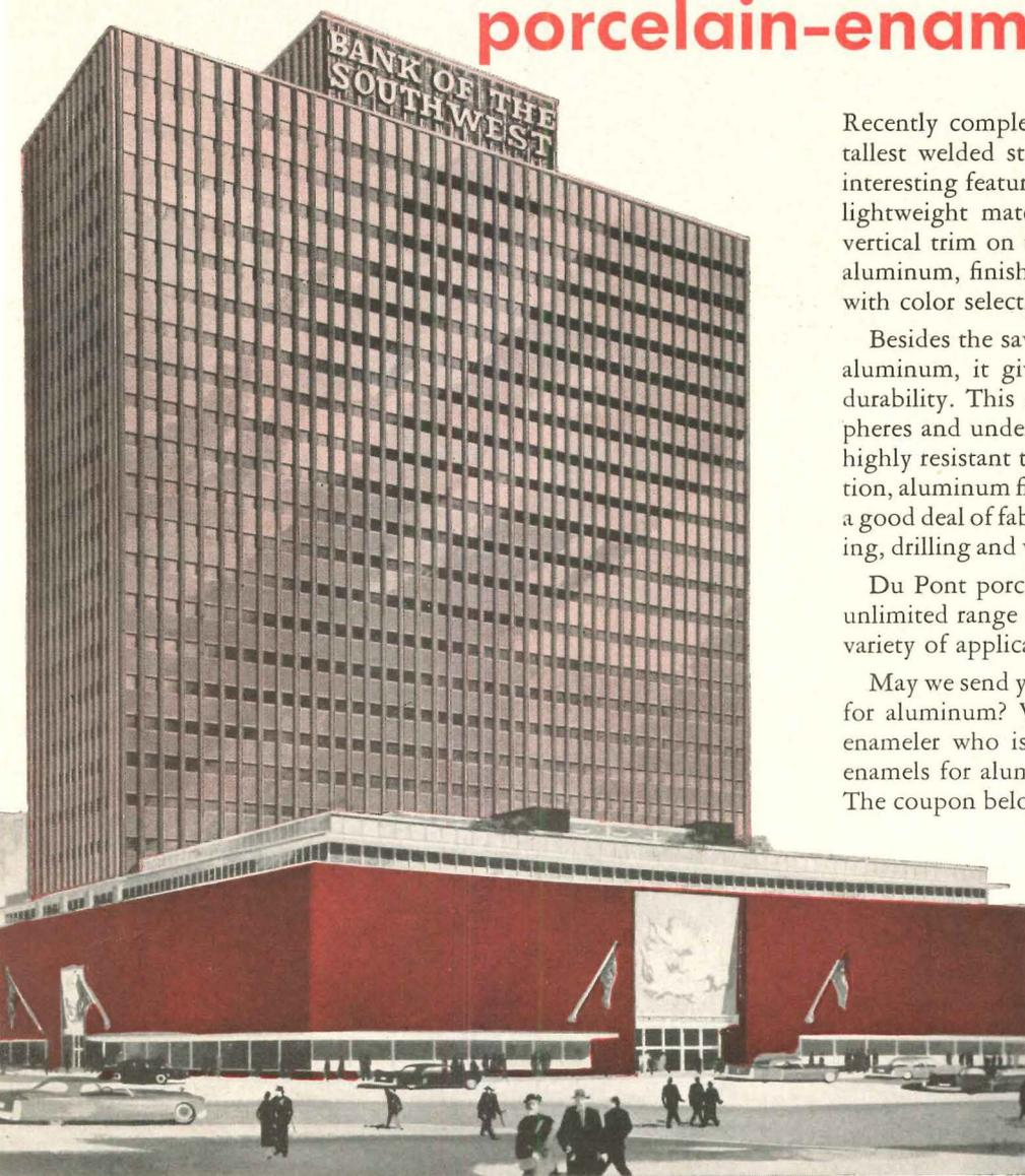
Recently completed, the Bank of the Southwest stands as the tallest welded structure in Houston, Texas. One of the many interesting features of this building is the extensive use made of lightweight materials in the superstructure—especially in the vertical trim on the mullion panels. Here, 32,892 linear feet of aluminum, finished with Du Pont porcelain enamel, were used with color selection to harmonize with the red granite base.
