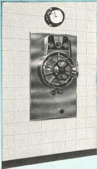
**THIS BUILT-IN CYLINDRICAL** pressure-type sterilizer is one of American Sterilizer Company's new units featuring "Cyclomatic Control." (See description in text.) Other features include welded, forged end ring of Monel, and sterilizing chamber, steam jacket, trays and slides of the same long-lasting, corrosion-resistant metal.
