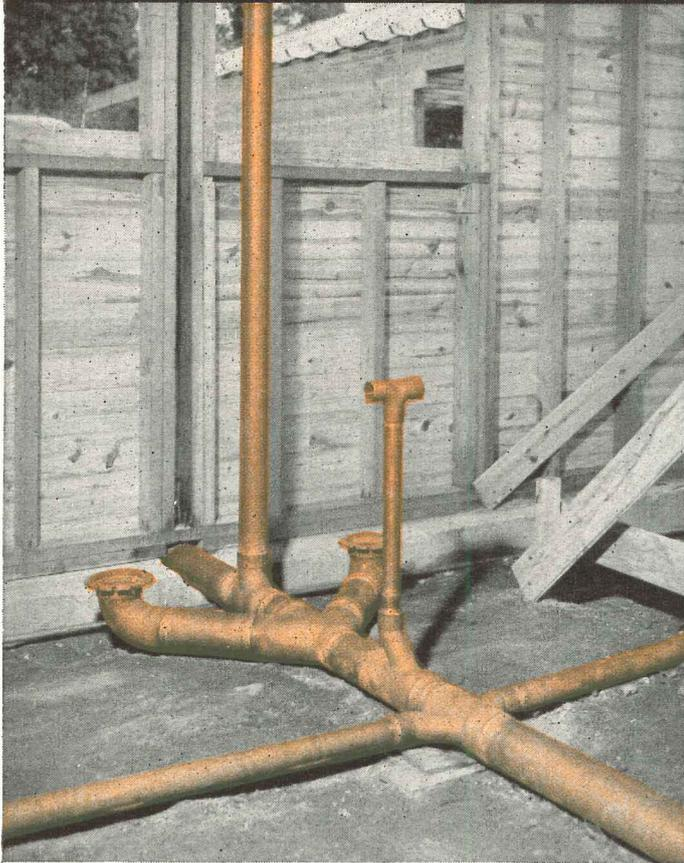
**ANACONDA** Type M Copper Tube and Fittings, in ranch-type residence under construction. Layout for two-bathroom arrangement. Includes 4" soil line; 3" vent stack; waste lines from bath tubs; waste line (riser) for lavatories.
