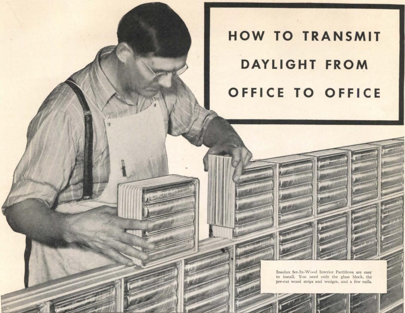
Insulux Set-In-Wood Interior Partitions are easy to install. You need only the glass block, the pre-cut wood strips and wedges, and a few nails.
