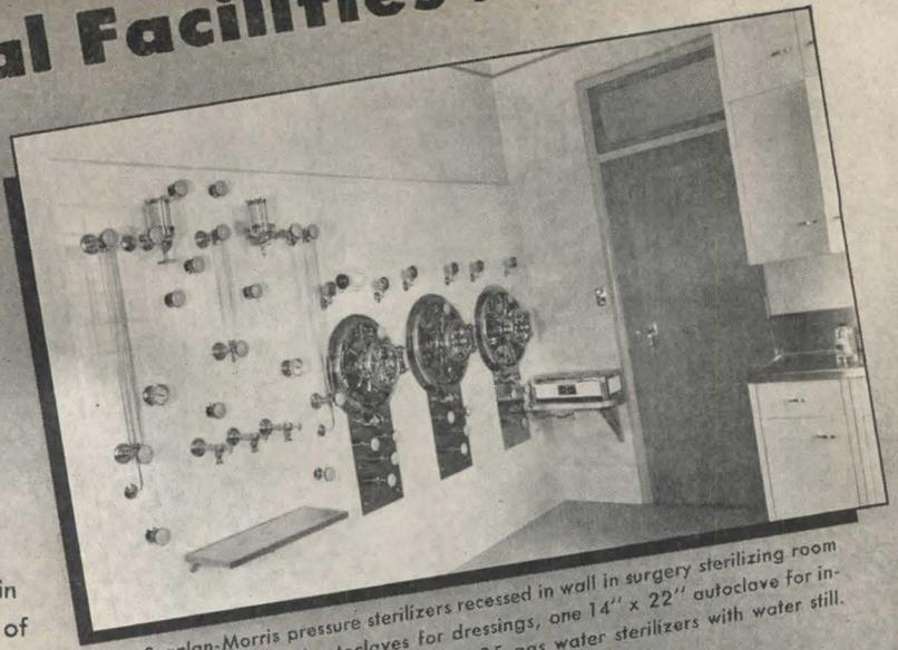
Scanlan-Morris pressure sterilizers recessed in wall in surgery sterilizing room—two 16" x 36" autoclaves for dressings, one 14" x 22" autoclave for instrument sterilization, and a set of 25-gas water sterilizers with water still.
