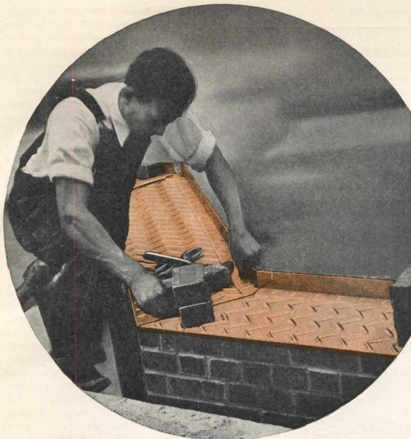
**Y**OU CAN READILY SEE from this illustration why Anaconda Through-Wall Flashing is known as "the flashing that drains itself dry on a level bed." The die-stamped dam and corrugations provide positive drainage in the desired direction, intercepting and disposing of wind-driven rain and moisture penetrating the masonry.
