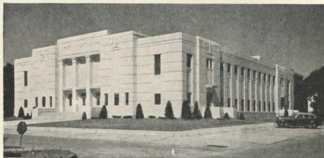
City Auditorium, York, Neb., designed by Meginnis & Schaumberg, architects, of Lincoln. Architectural concrete details produced by use of milled wood and plaster molds. Smooth exterior concrete walls cast in plywood forms.
