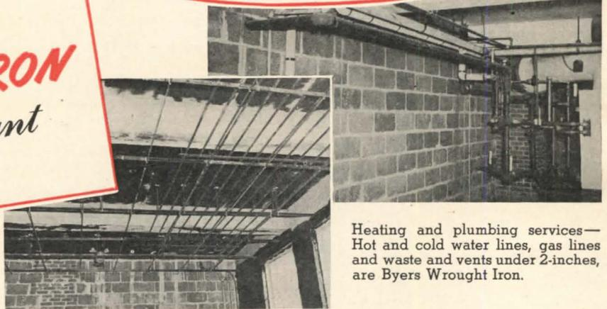
Radiant Heating Coils of Byers Wrought Iron are installed in first floor construction and ceilings.
