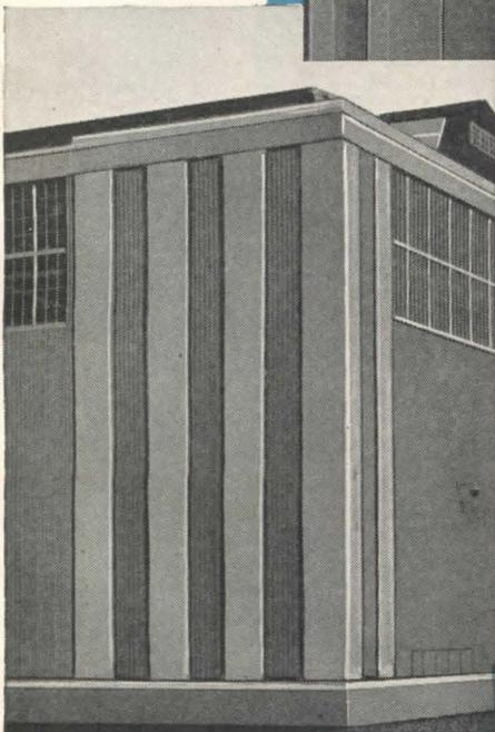
Typical Exterior, Mahon Steel Deck Sidewall Construction. Pilaster effect is obtained by reversing Deck Plates so that ribs face in, as opposed to remainder of wall where ribs face out.
