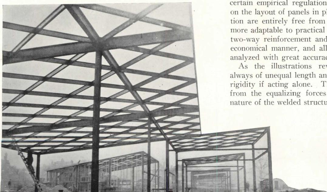
Fig. 1. Structures framed with the "Dia-Grid" system
