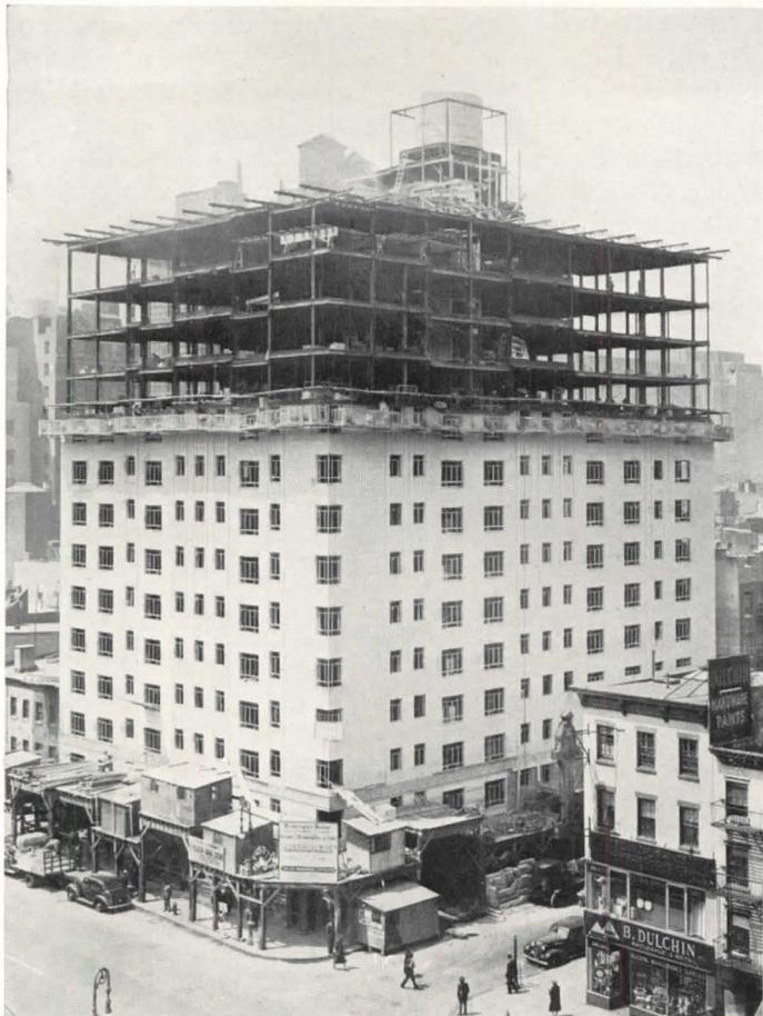
Fig. 15. A welded-frame apartment house recently completed in New York—first American city to amend its building code to permit welding.
