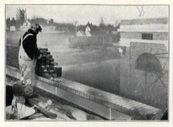
Cheney Flashing installed in Parapet wall. Note keys ready for mortar to form "The Unbreakable Key Bond"
