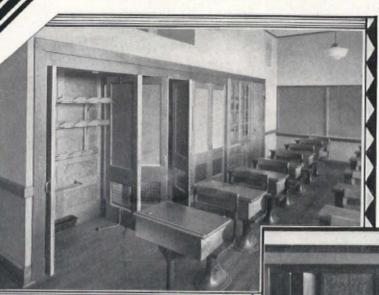
Showing installation in class room of Belmont, Mass. High School. Note how doors do not block aisle when wardrobe is open.
