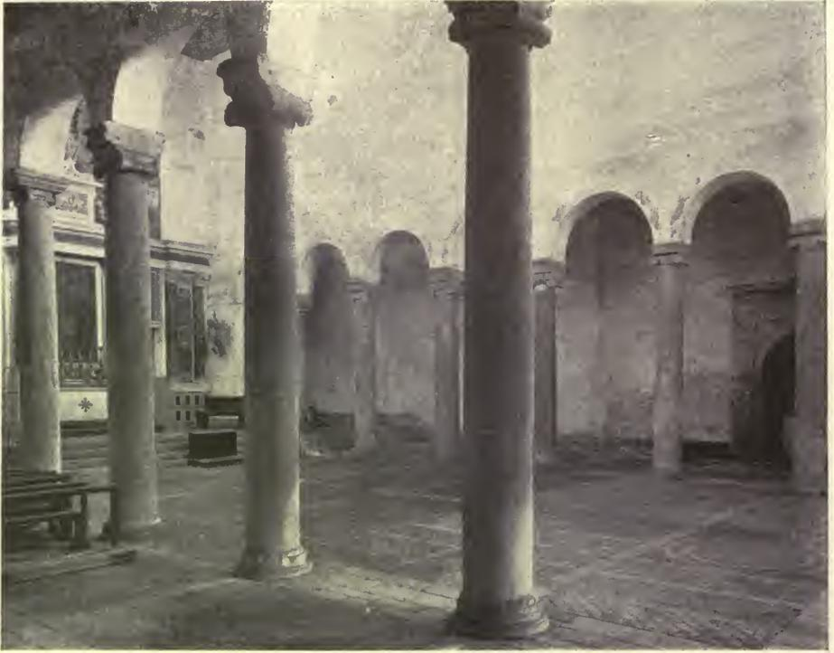
FIG. 25.—THE SLOPING PAVEMENT OF S. SABA AT ROME.
