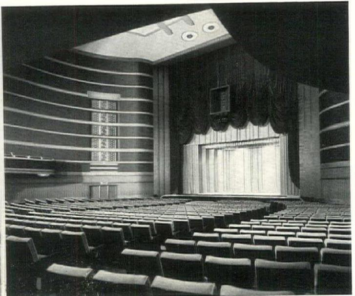
Kansas City Auditorium. Left: seats laid out in curved rows provide a maximum of comfort for spectators besides reducing wear on upholstery and strain on seats. Right: use of curved aisles introduces automatic staggering of seats without destroying alignment at aisles. Use of fully upholstered seats reduces acoustic problems
