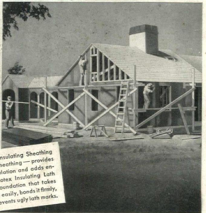
Celotex Vapor-Seal Insulating Sheathing replaces ordinary sheathing — provides moisture-proofed insulation and adds enduring strength. Celotex Insulating Lath provides a strong foundation that takes plaster smoothly and easily, bonds it firmly, and permanently prevents ugly lath marks.
