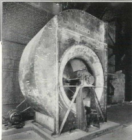
One of 14 Sturtevant Fans supplying 980,500 c.f.m. of fresh air, 2200 tons per hour.
