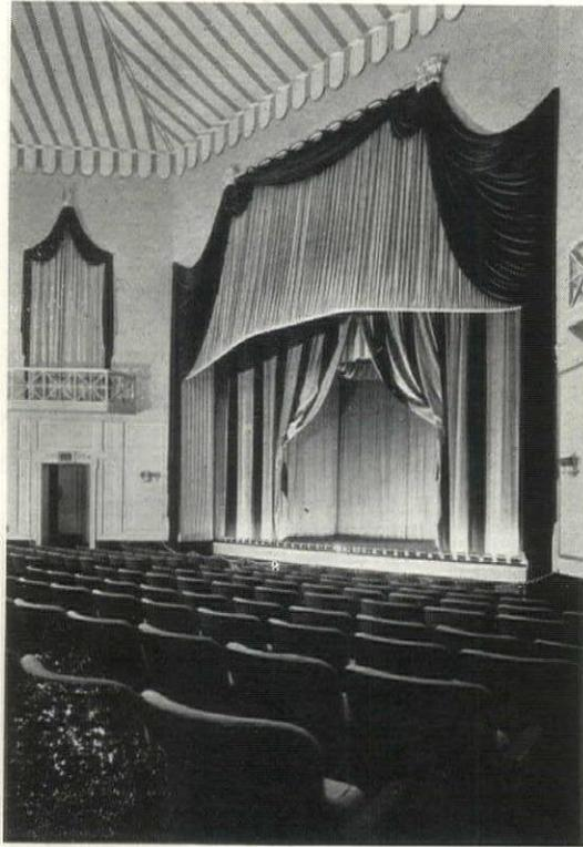
An excellent illustration of the automatic staggering of seats at the front of the theater which is produced by the use of a fan-shaped plan
