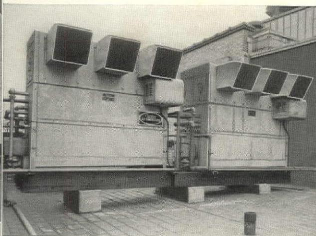
**... CARRIER EVAPORATIVE CONDENSERS** were located on the roof. Using less than 5% of the water required by water condensers or other type of water equipment, these efficient condensers solved the Leader Building's problem completely, without enlarging water mains.
