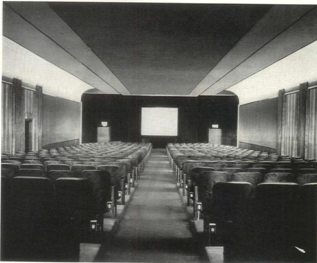
The single aisle down the center of this cinema eliminates what would ordinarily be the best seats in the house. Seats are laid out in straight rows from front to back; there is no staggering. To partially overcome difficulties of horizontal sight-lines, pitch of floor has been increased using risers at the rear
