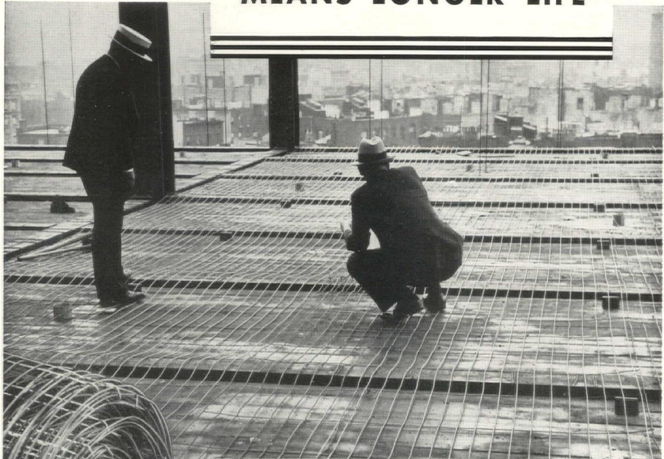
**C**ONCRETE walls, floors and roofs are stronger and last longer if the concrete has been reinforced with wire fabric.
