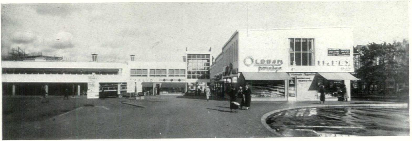
The structure consists of reinforced concrete frame with light weight brick, cork, heraclith and insulite used as fill and insulation. Exterior surfaces are finished with a very thin coat of plaster and painted white. The large restaurant (below) is located on the second floor and runs almost the entire length of the building
