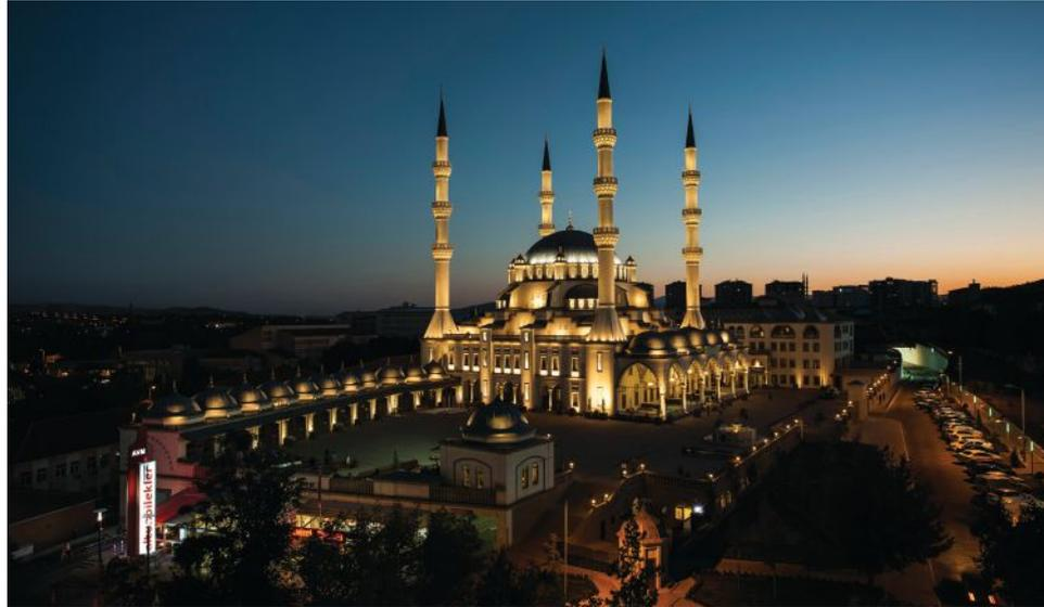
Zeve Lighting used short-throw, narrow-beam luminaires to accentuate the high-relief patterns of muqarnas, a form of high-relief honeycomb-like vaulting, above the columns. Wide-beam fixtures bathe the undersides of the entry dome with warm-white light, and a warm-white spotlight demarcates the main entrance. Where possible, fixtures were concealed or painted to match or minimize their daytime visibility.
