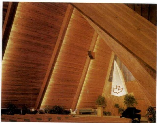
Indirect ambient light, supplied by linear fluorescents concealed in floor-to-ceiling coves, illuminates the interior of the chapel with a warm, rich glow. The system can be dimmed to various settings to accommodate the variety of activities that occur in the space.
