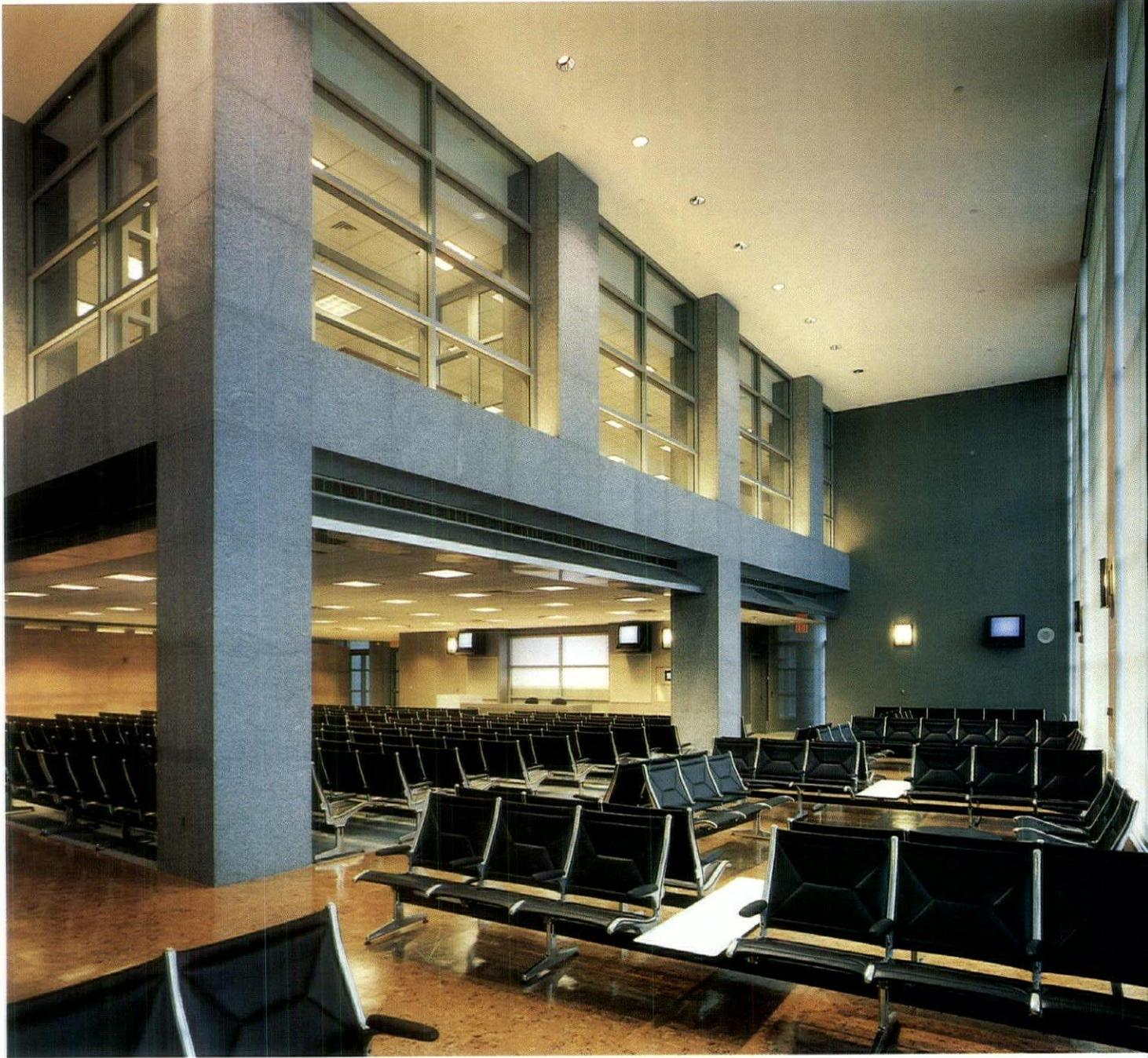
FLUORESCENT UPLIGHTS IN THE TROUGHS AT THE BASE OF WINDOWS IN THE JURY ASSEMBLY ROOM (ABOVE) PROVIDE AMBIENT LIGHT. CEILING-RECESSED METAL HALIDE DOWNLIGHTS PROVIDE READING ILLUMINATION AND COMPACT FLUORESCENT WALL SCONCES OFFER HUMAN SCALE.
