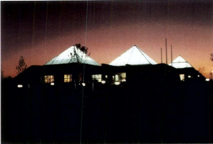
**CHALLENGE** The facility is divided into three spaces, each defined from the outside by a pyramidal roof made of a translucent material, designed to glow at night when illuminated from inside.
