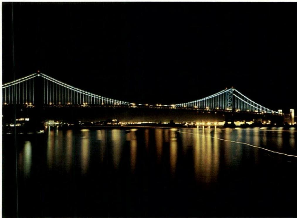
*Award of Excellence winner. The lighting scheme for the Benjamin Franklin Bridge emphasizes the main catenary cables and vertical suspender cables that support the bridge deck. Computer-generated animation patterns are triggered by trains crossing the bridge.*
